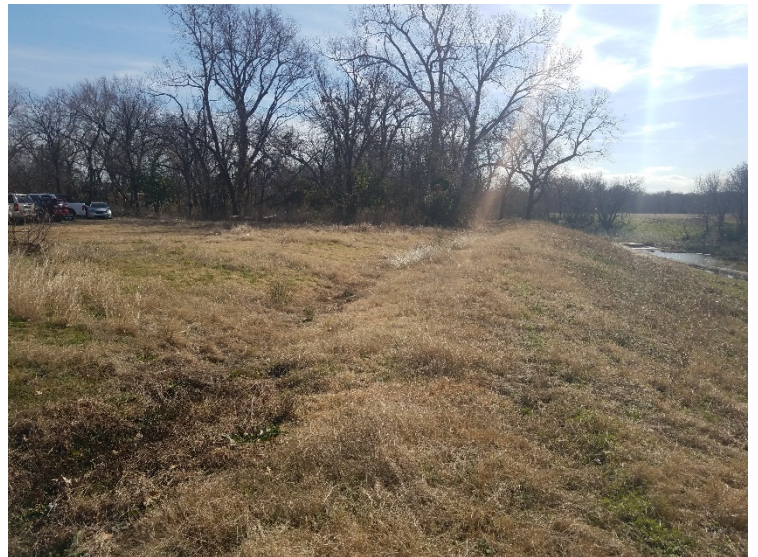
Photograph 12 – Graded creek bank within Northern APE, view to the southeast.
