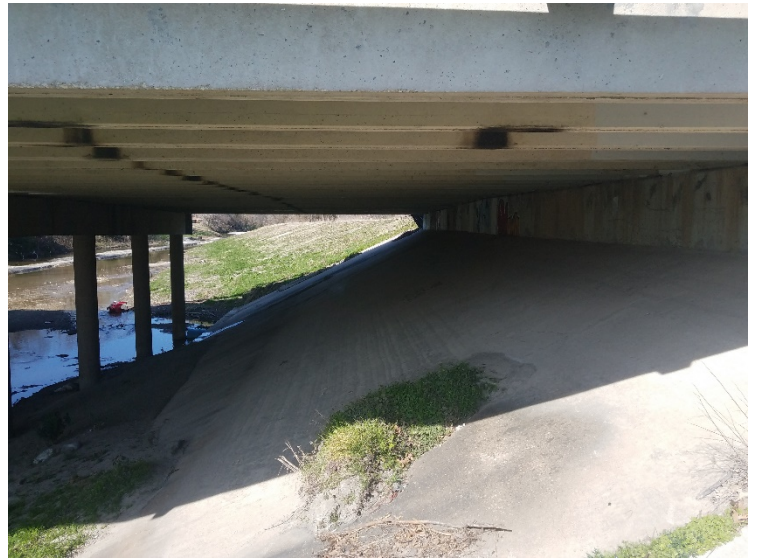
Photograph 10 – Northern APE passing under Centerville Road bridge, view to the northwest.
