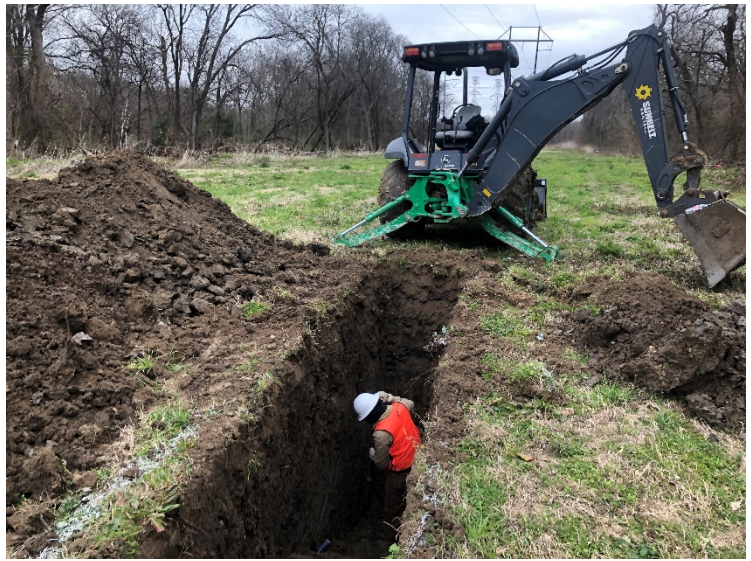
Photograph 24 - Trench 1 within Southern APE, view to the southeast.
