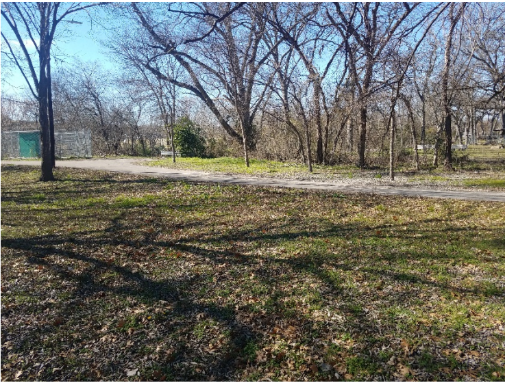
Photograph 15 - Stormwater outflow processing structure and concrete sidewalk within Northern APE, view to the southwest.
