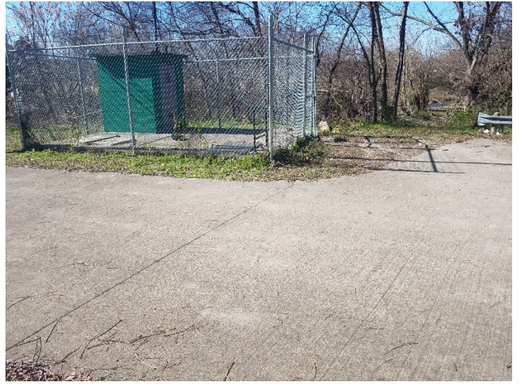
Photograph 14 - Stormwater outflow processing structure and concrete sidewalk within Northern APE, view to the southwest.
