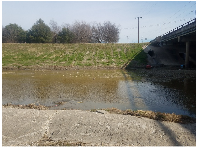
Photograph 4 – Location of pedestrian bridge within Northern APE with graded creek bank, view to the northeast.
