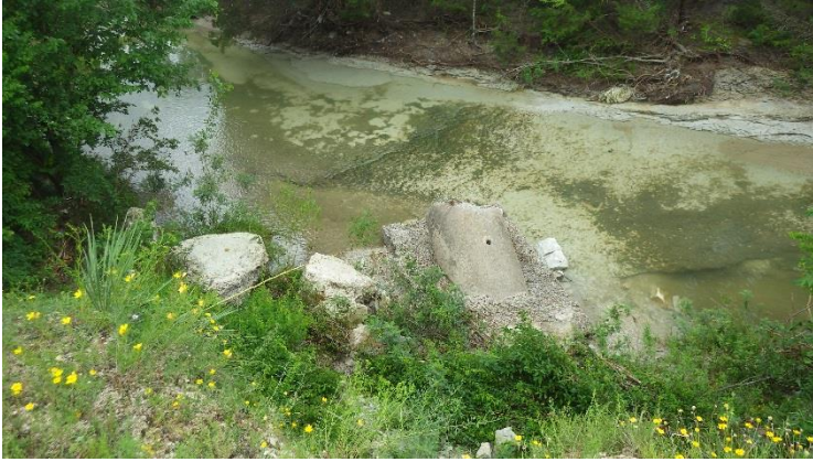
Photograph 25 – Debris in channel from bank erosion, view to the southwest.
