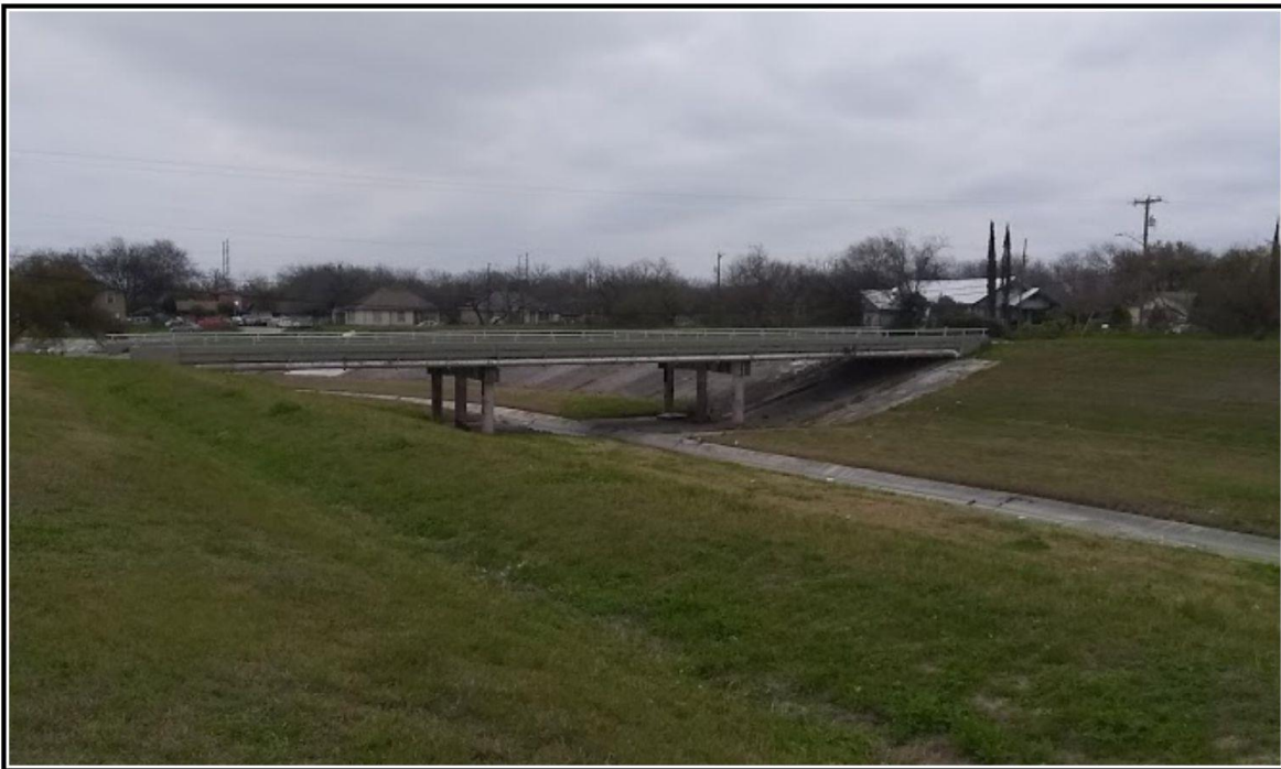
Figure 2-1. Zarzamora Creek facing northeast towards Fortuna Street bridge.
