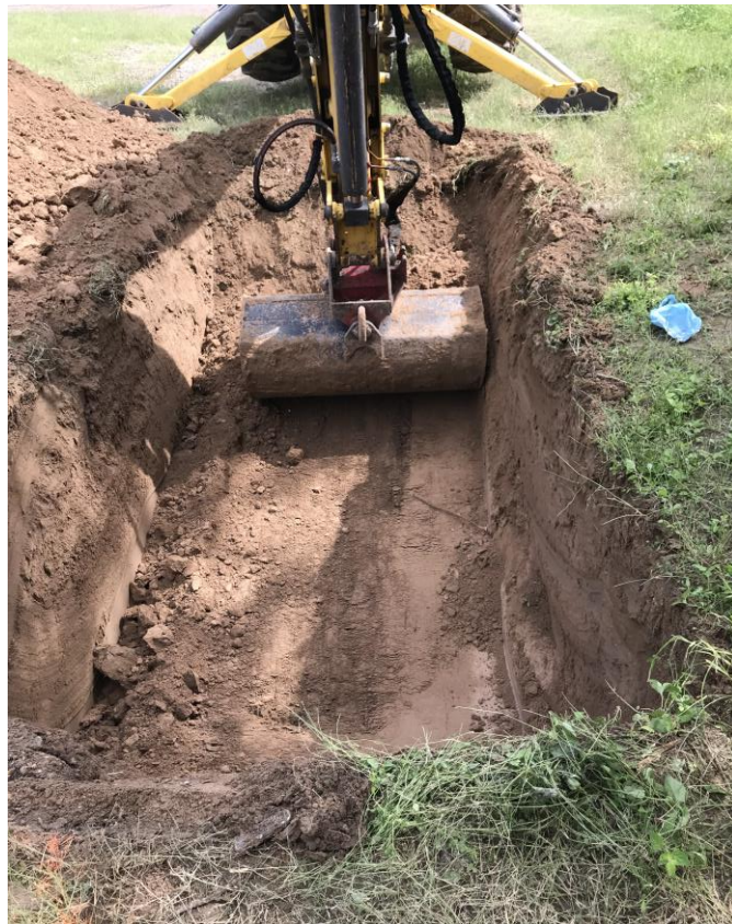
Trench 2 scraping on US 83 ROW near Roma Cemetery (looking west).
