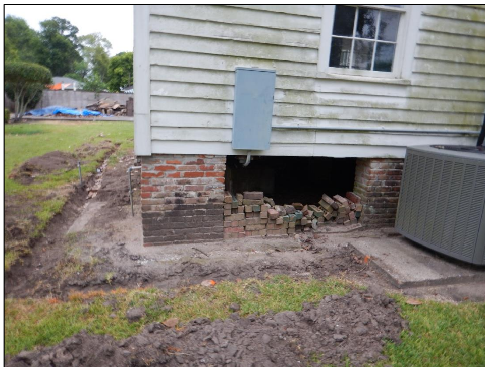
Figure 5-12. Northern section of the western and northern trenches. Note stacked brick between piers.
