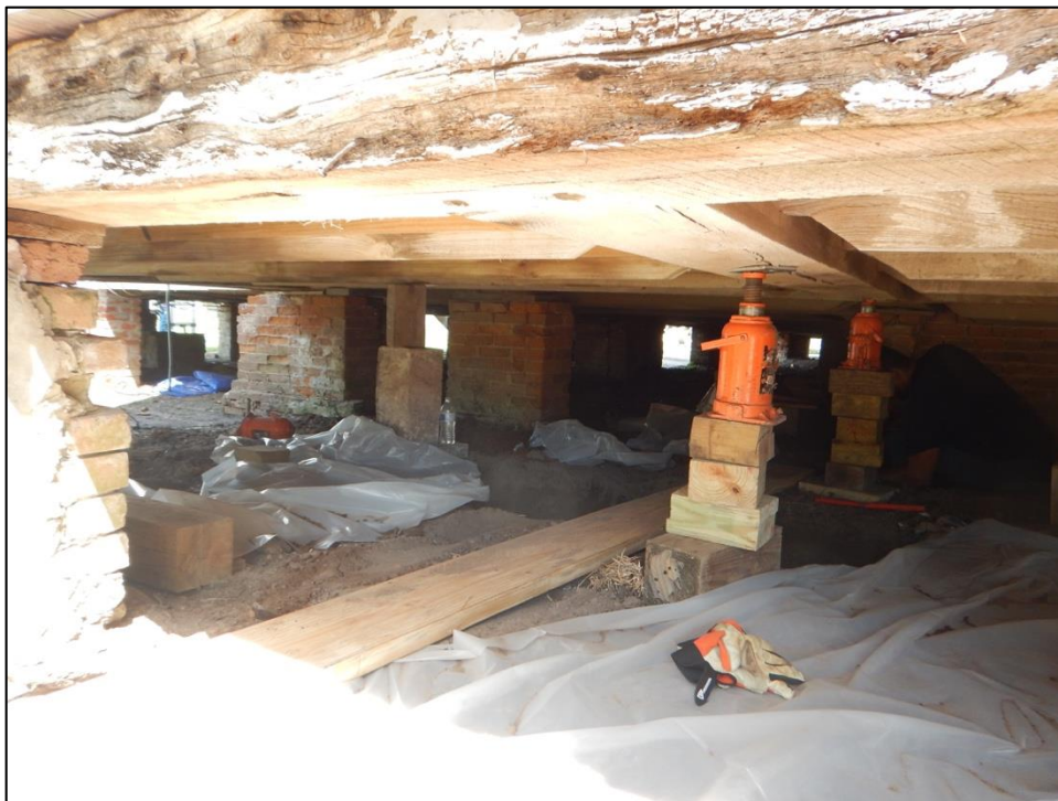
Figure 5-15. Temporary piers and plastic located in the crawl space as piers were excavated.
