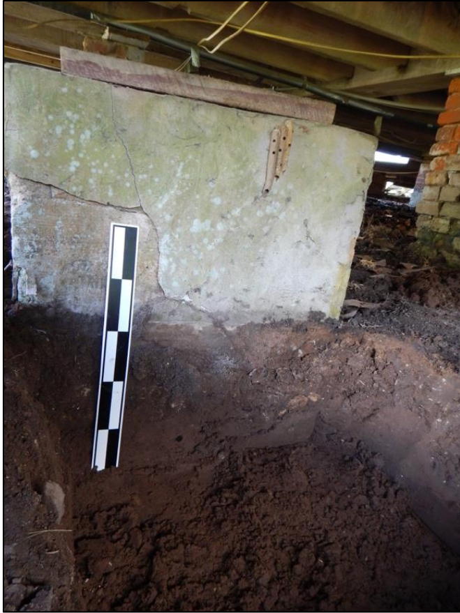
Figure 5-19. Pier excavated adjacent to the well. Soils were saturated.
