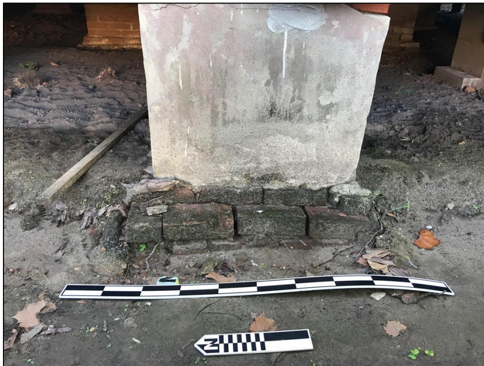
Figure 5-14. Typical pier on the western side of the house, showing brick footing exposed by trench.
