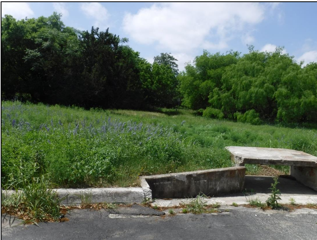
Figure 5-12. Overview of Location 3, facing southwest.
