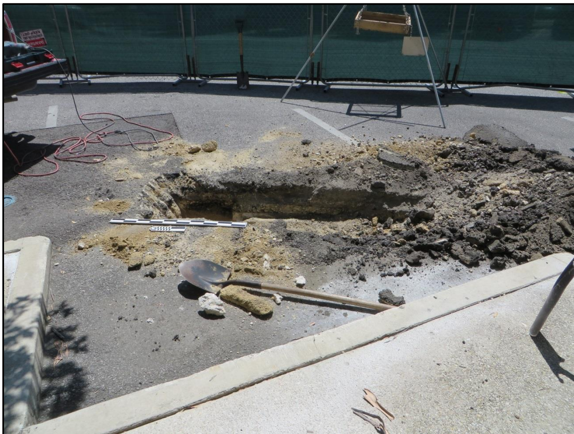
Figure 4-2. The RKEI exploratory trench in Phase I.
