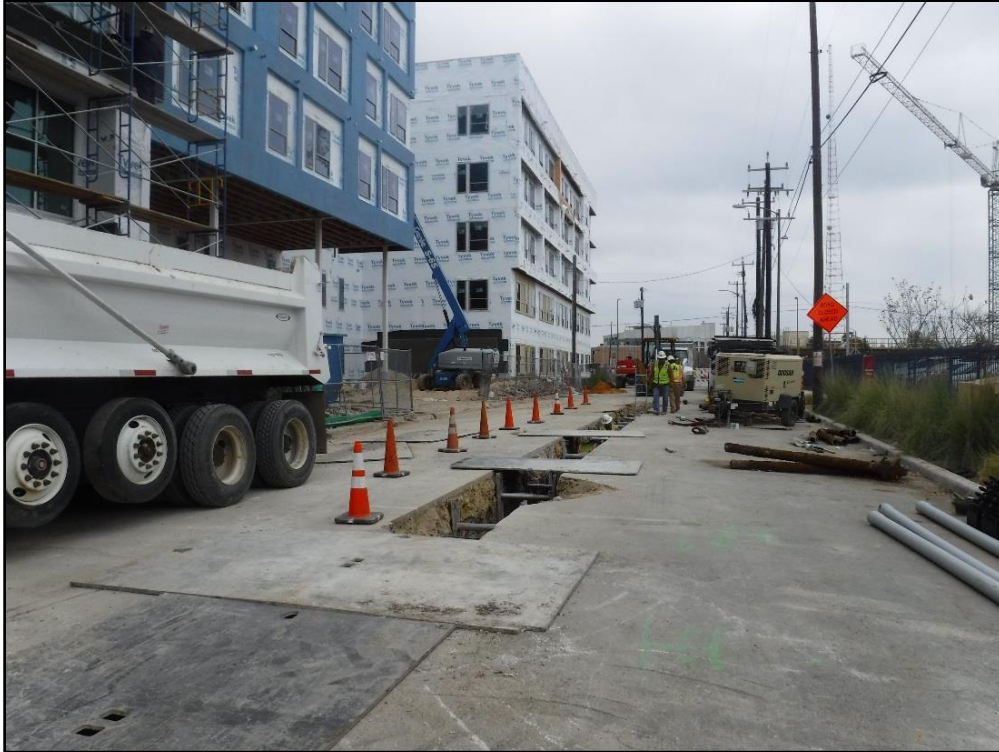
Figure 5-2. Overview of the APE excavations, facing east.
