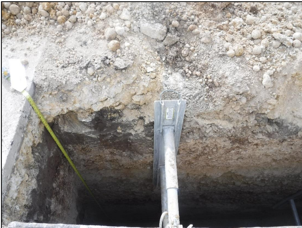
Figure 5-5. Average soil profile for manhole pit excavations, facing south.
