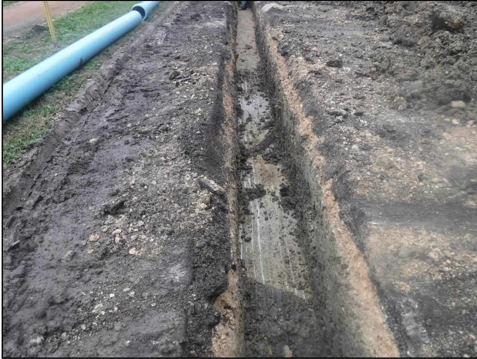
Figure 5-14. Modern concrete slab observed within the extended APE monitoring area, facing west.
