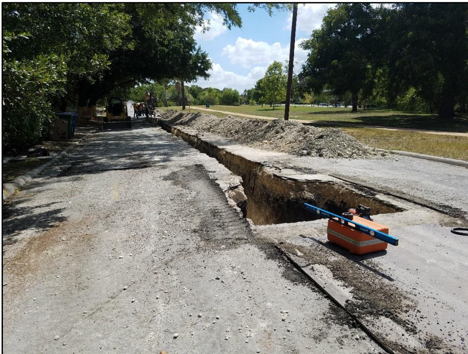
Figure 5-4. Overview of sewer main installation excavations within the APE, facing southeast.
