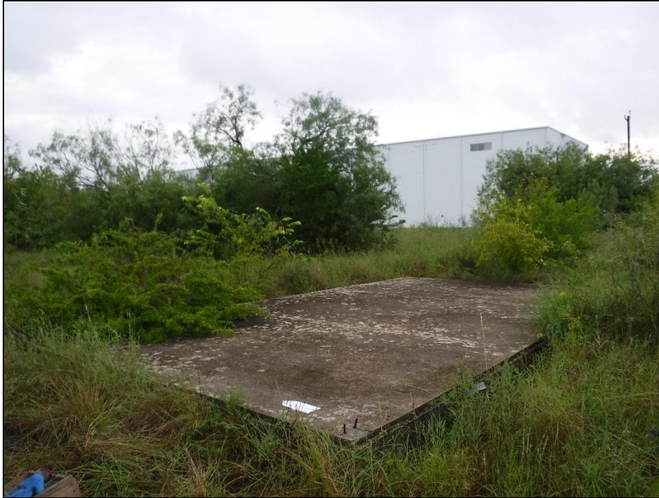
Figure 5-9. Cement Pad 3, facing northeast.
