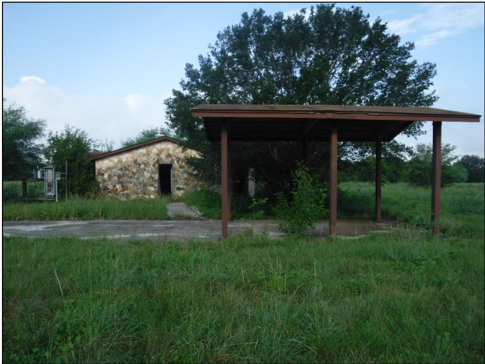
Figure 5-3. Covered concrete slab, facing west.
