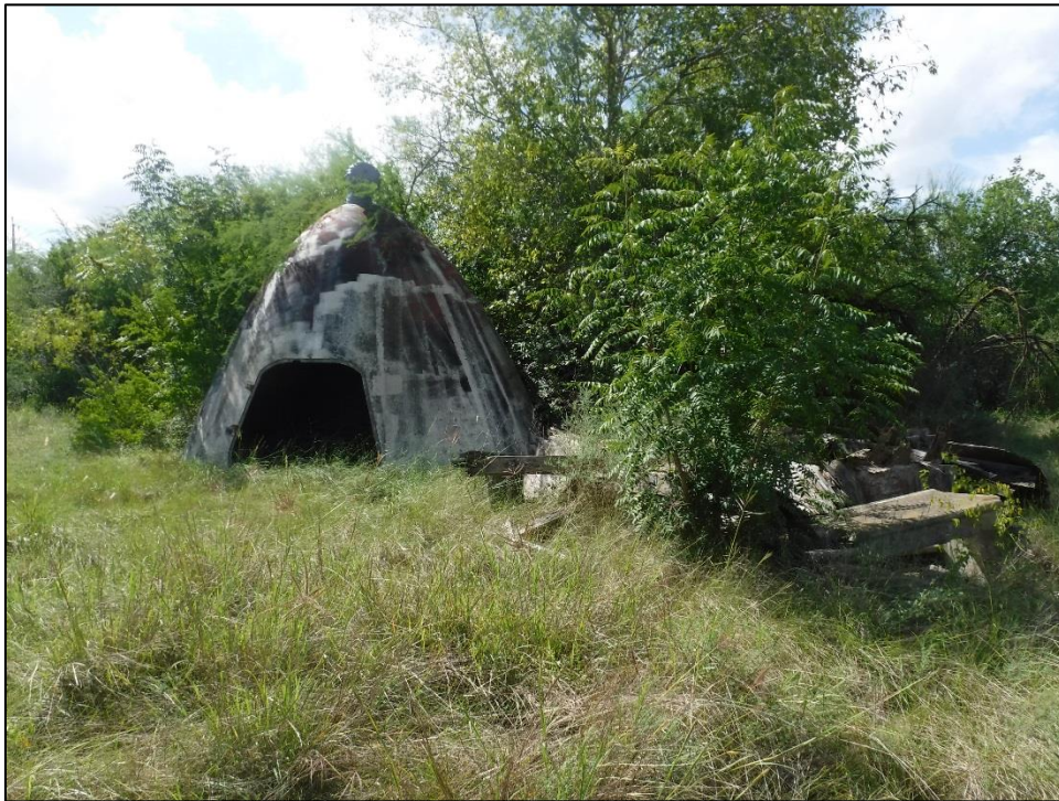
Figure 5-5. Aircraft nosecone huts, facing southwest.
