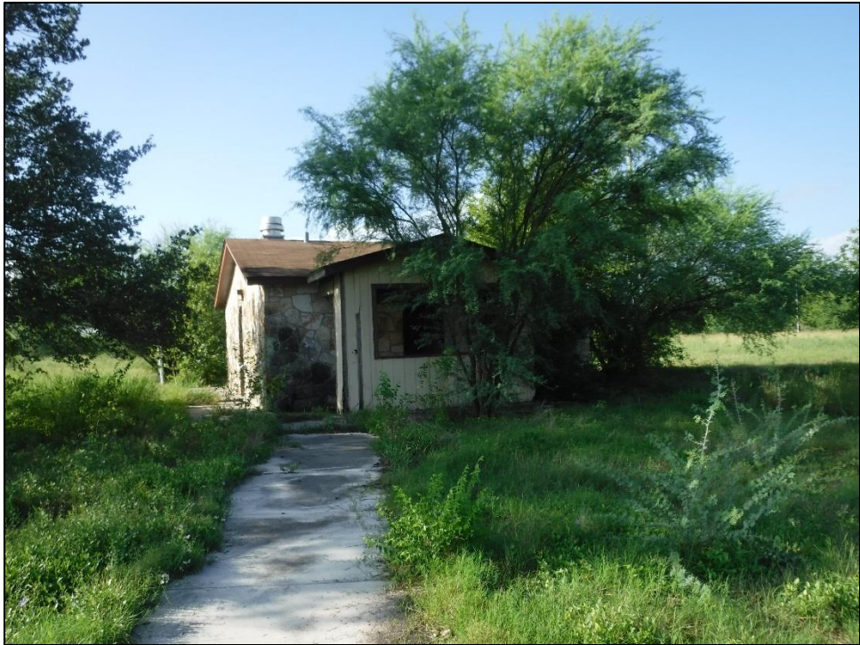
Figure 5-2. FamCamp Restroom and Showers, facing north.
