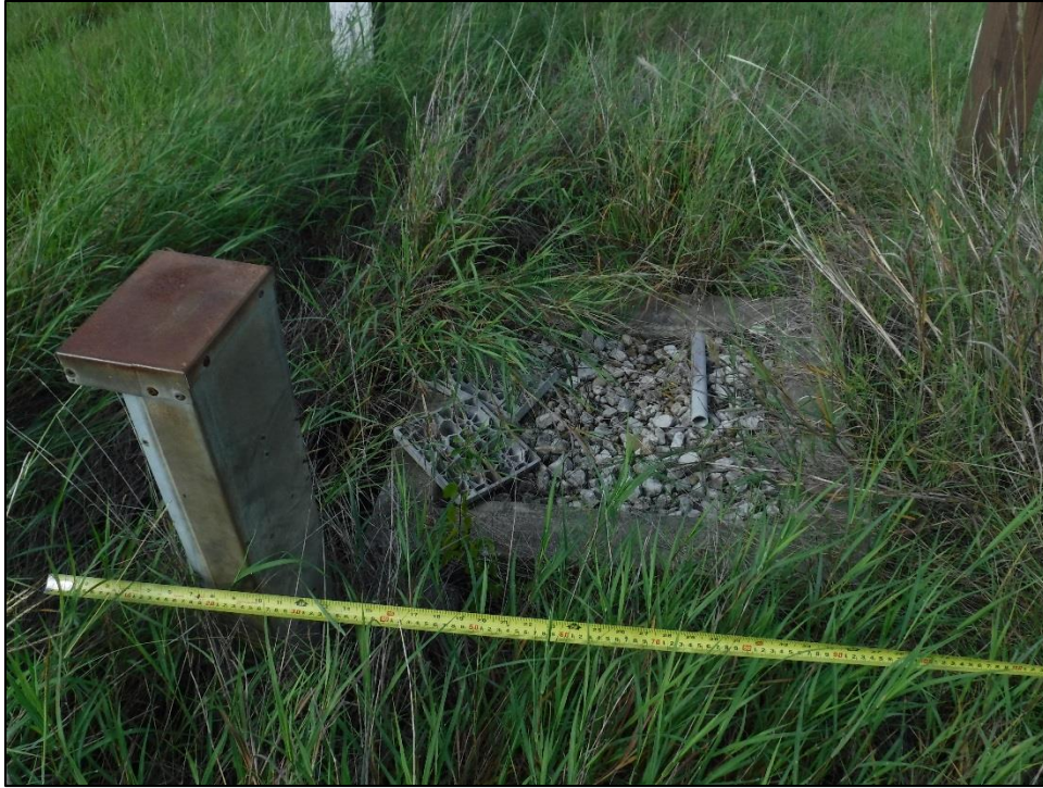
Figure 5-4. R.V. Hookup, facing north.
