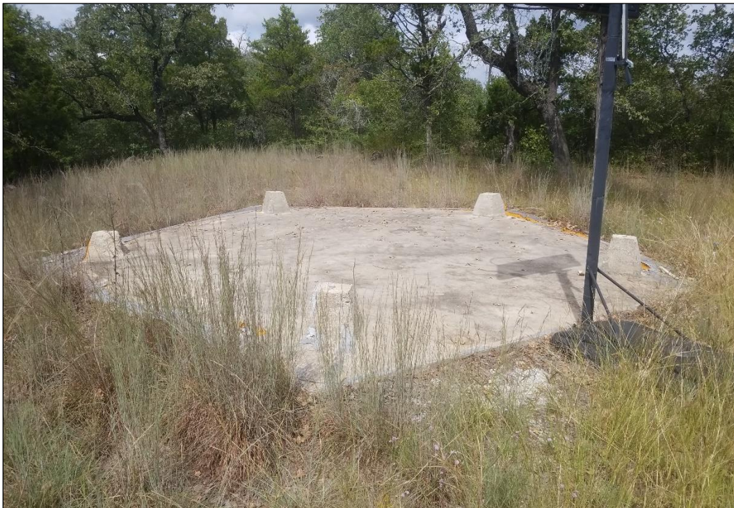
Figure 19. Concrete Basketball Court North of Eastern Residence (Facing Northeast)
