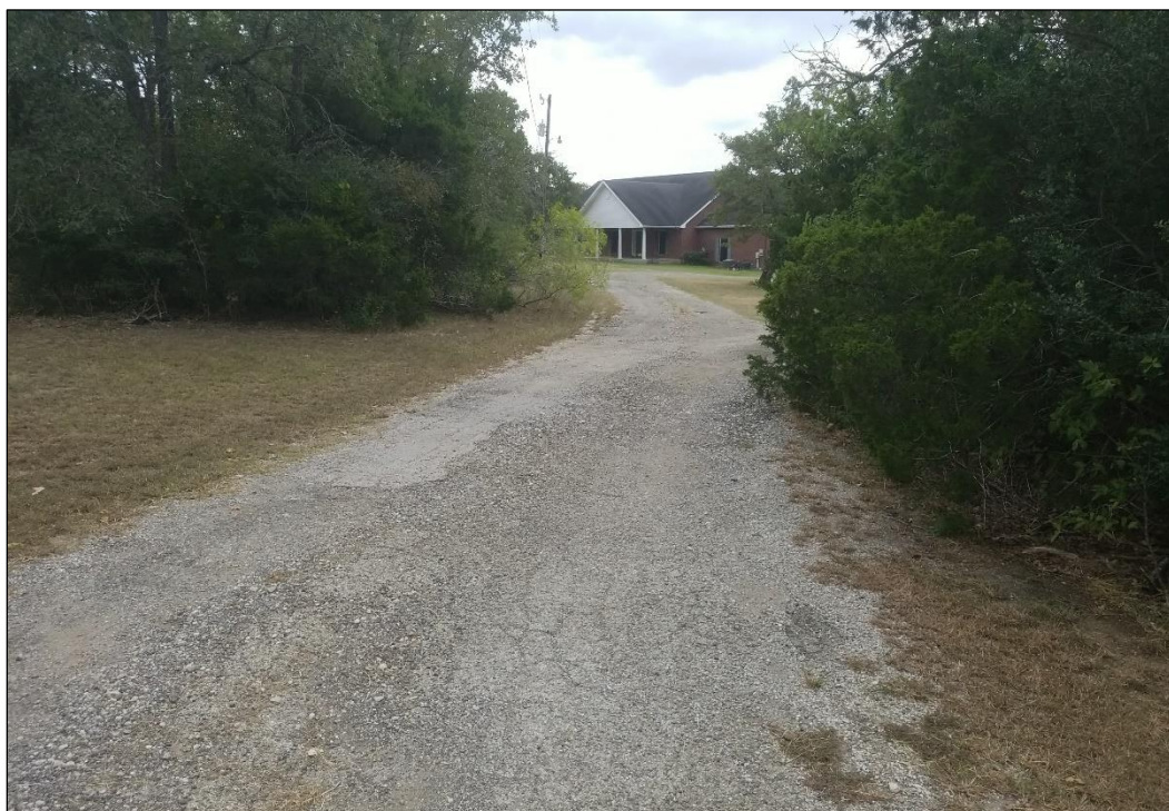
Figure 11. View of Modern Western Residence and Asphalt Driveway (Facing Southeast)
