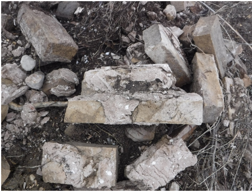
Figure 8. Representative bricks with mortar.
