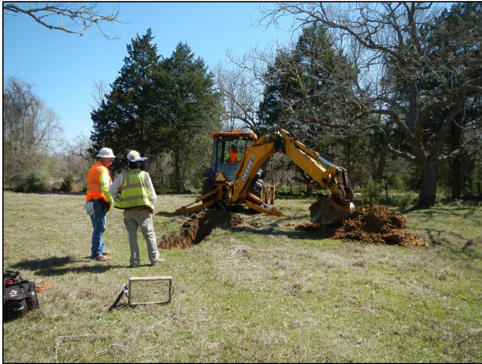
Figure 6. Backhoe trench BHT02 overview, facing east.
