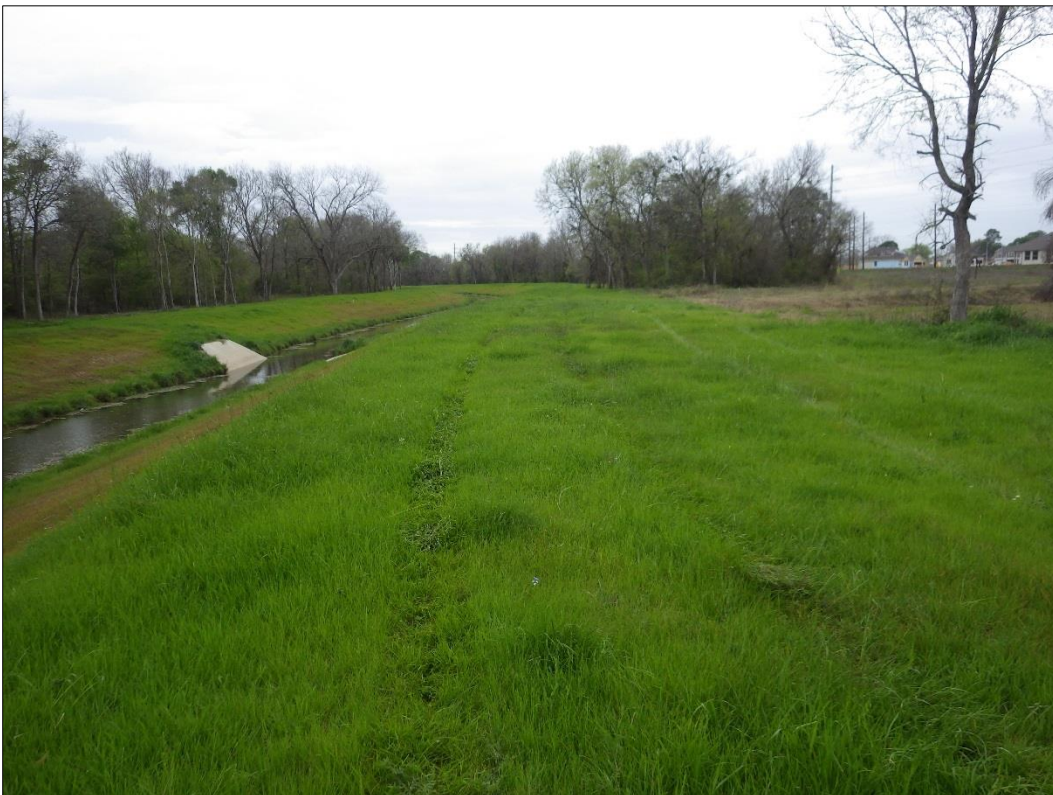
Figure 7. Channelized Seabourne Creek showing maintained creek bank.
