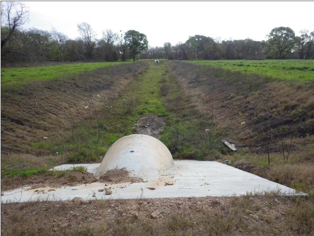
Figure 6. Excavated drainage ditch through Parcel 1.
