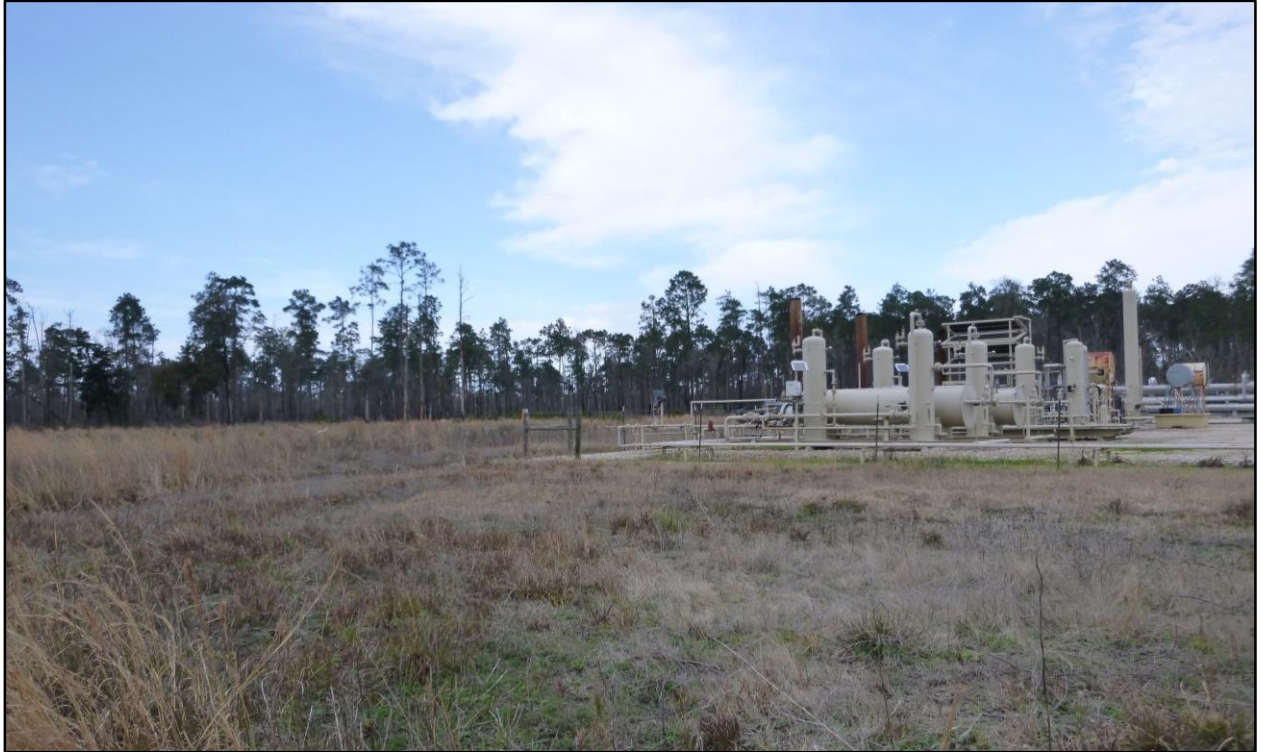
Figure 4. View of the western well pad location, west.
