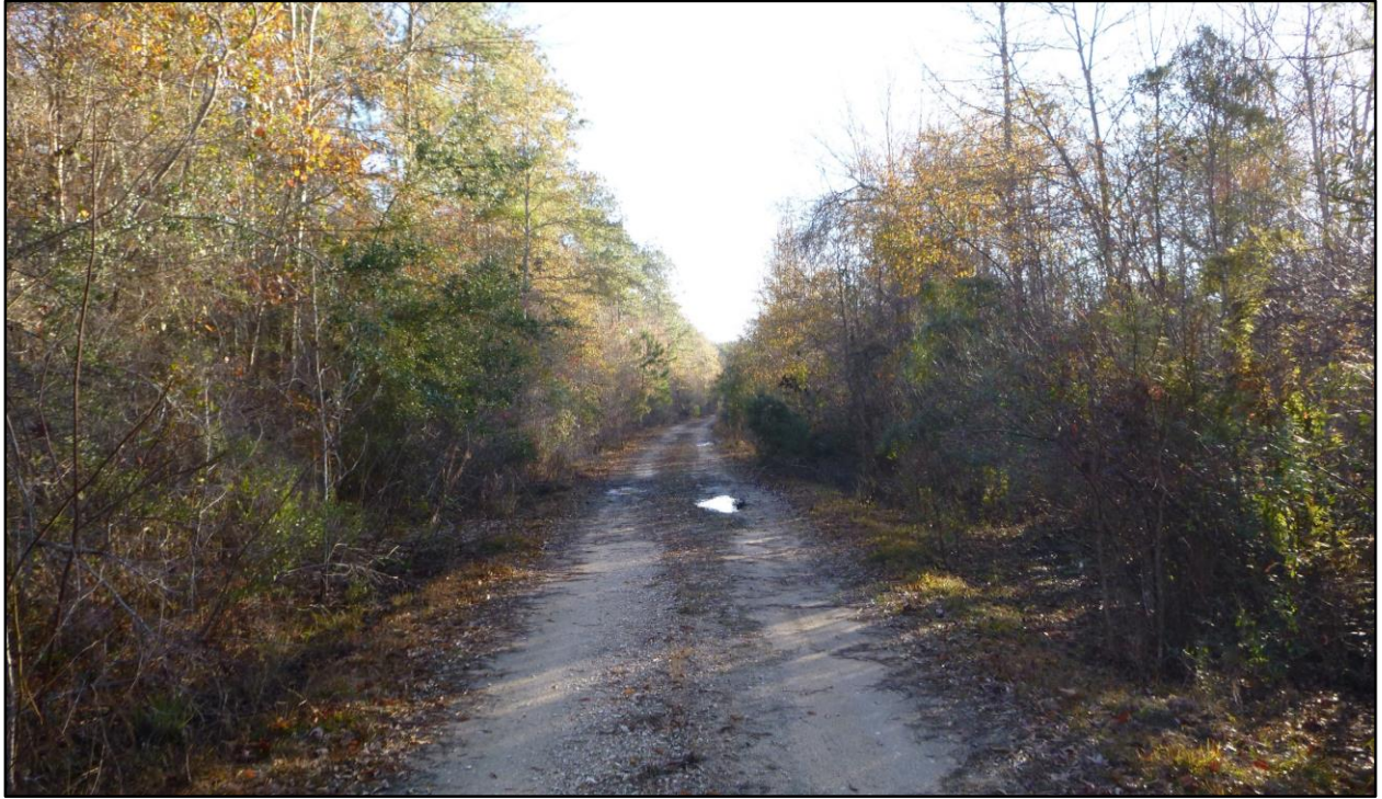
Figure 8. View of proposed pipeline line corridor to the right of the road, facing east.
