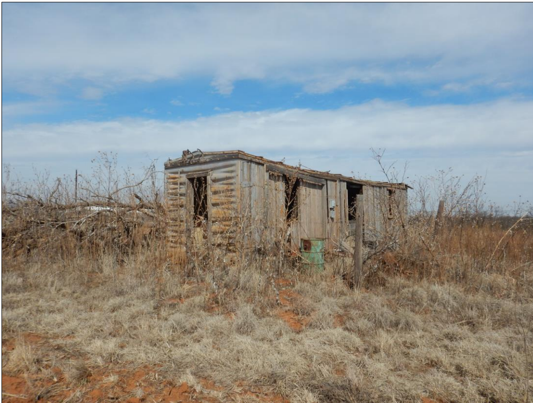
Figure 23: Railroad train car that has been converted to a storage shed.
