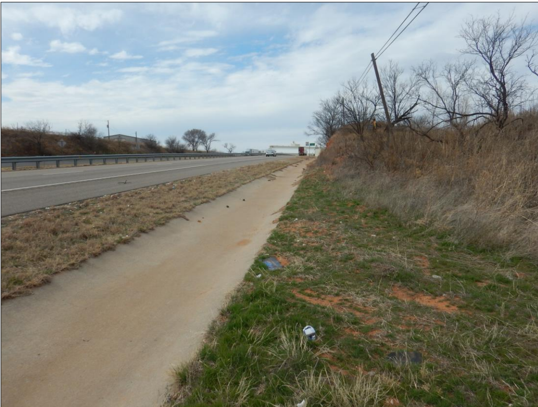
Figure 17: Concrete drainage ditch north of US 287.
