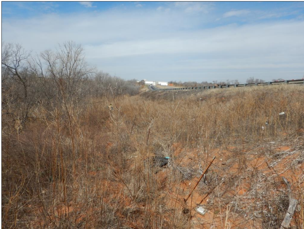
Figure 11: Fence line separating new and existing ROW with overgrowth vegetation
