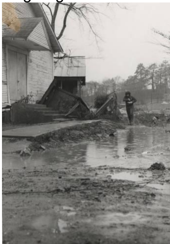
Figure 5: Church and house in Little Creek Community after the flood (ETRC). According to Boris Caldwell (Facebook post) the structure in the forefront was a church and the other building pictured was Lora Hunt Woodson's house (his great grandmother).
