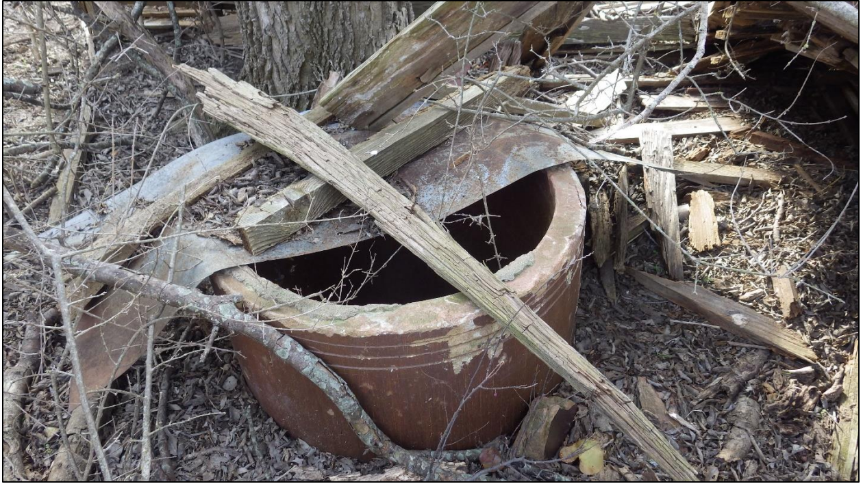
Figure 12. Water feature (cistern or well) at the northeast corner of the collapsed structure in 41COL328.
