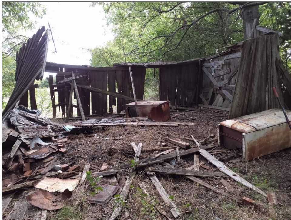
Figure 37. Detail of Structure 1 at 41COL338, facing south.
