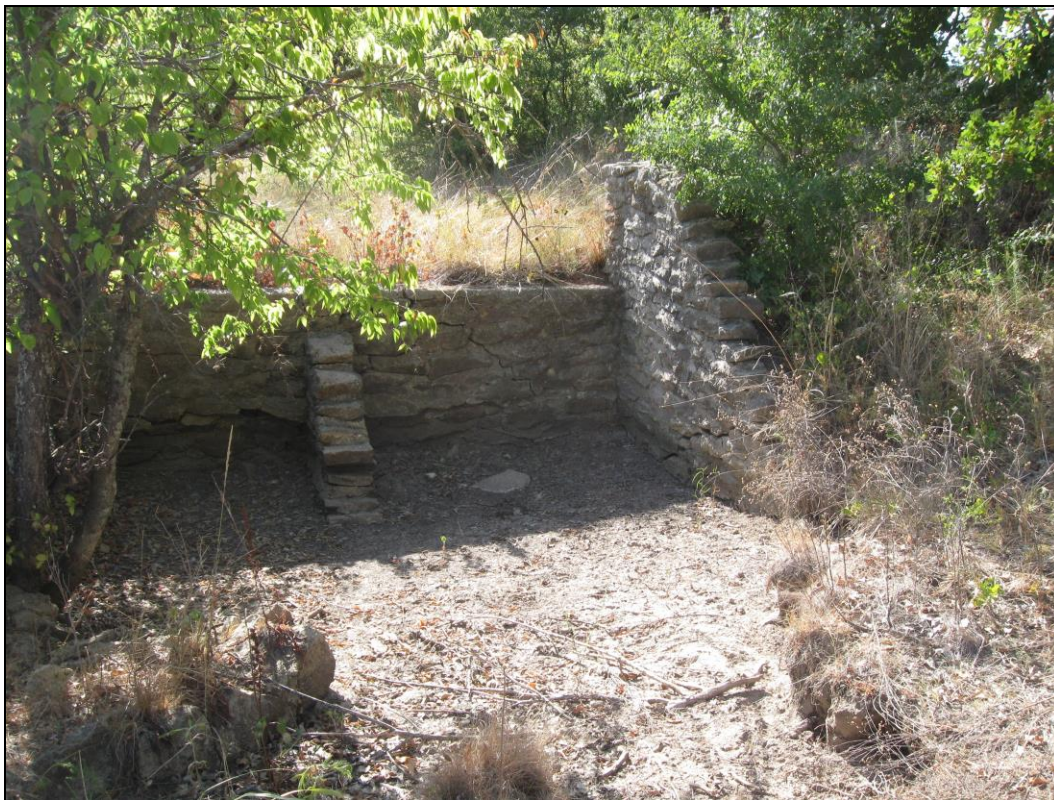
Figure 12. Representative view of the stone and concrete soil erosion control structures
