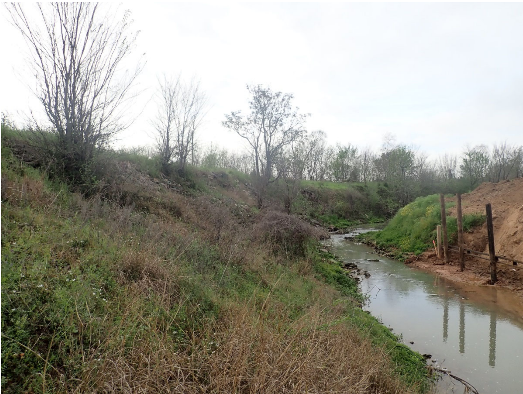
Figure 5-6. Overview of riprap along channelized bayou and Site 41FB102 centroid. View is facing southeast.
