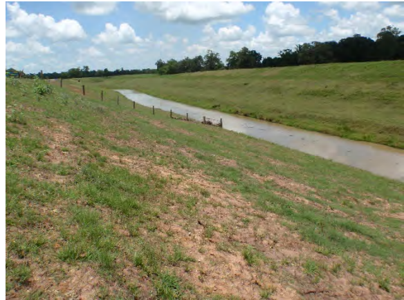
Figure 5-13. Overview of Workspace 4 APE. View is to the north.
