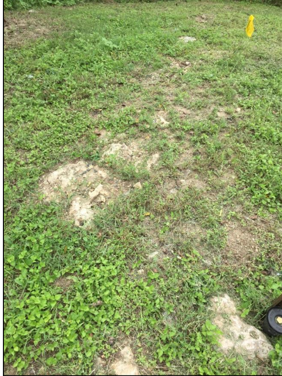
Figure 18. Shallow, exposed bedrock on ROW, east of Great Oaks Drive Bridge.
