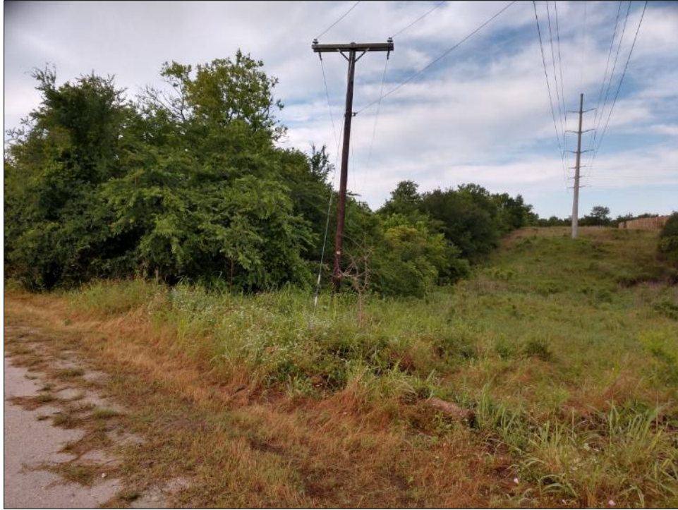
Figure 19. Steep slope on inaccessible property 70187.
