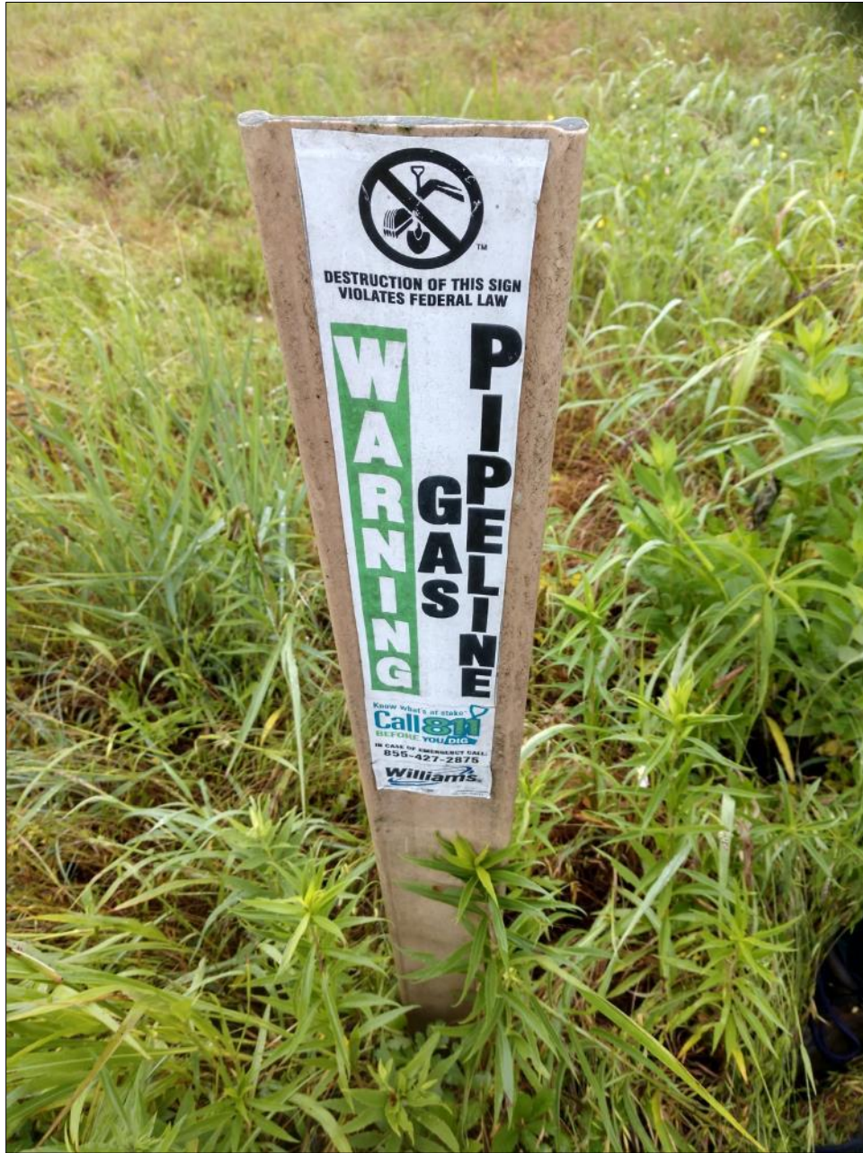
Figure 18. Gas line in Disturbed Area 3.
