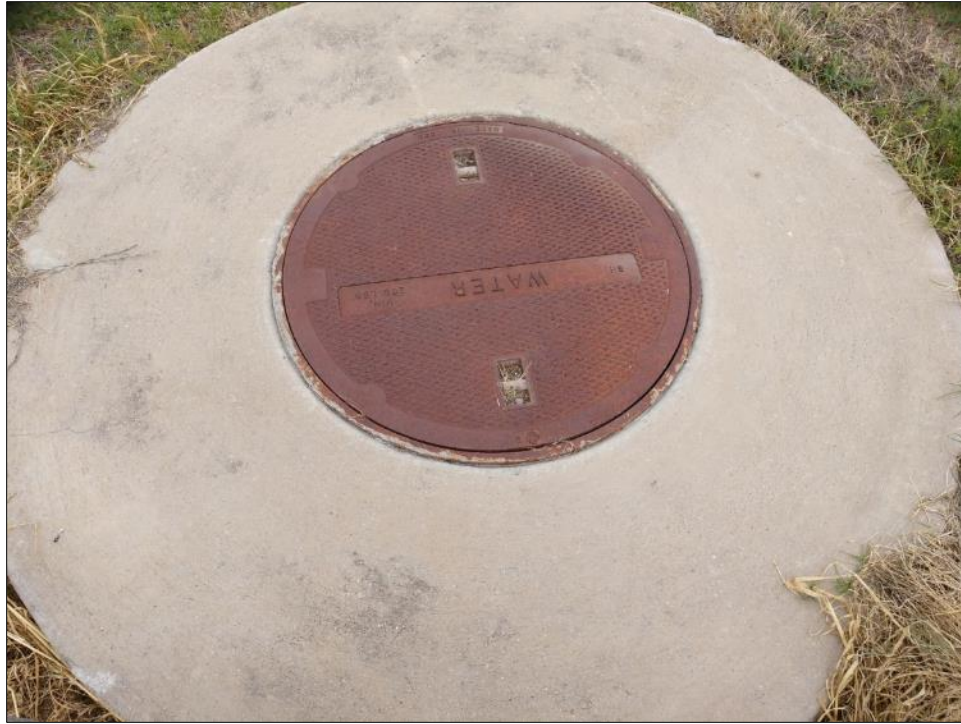
Figure 10. Water line within Disturbed Area 1.
