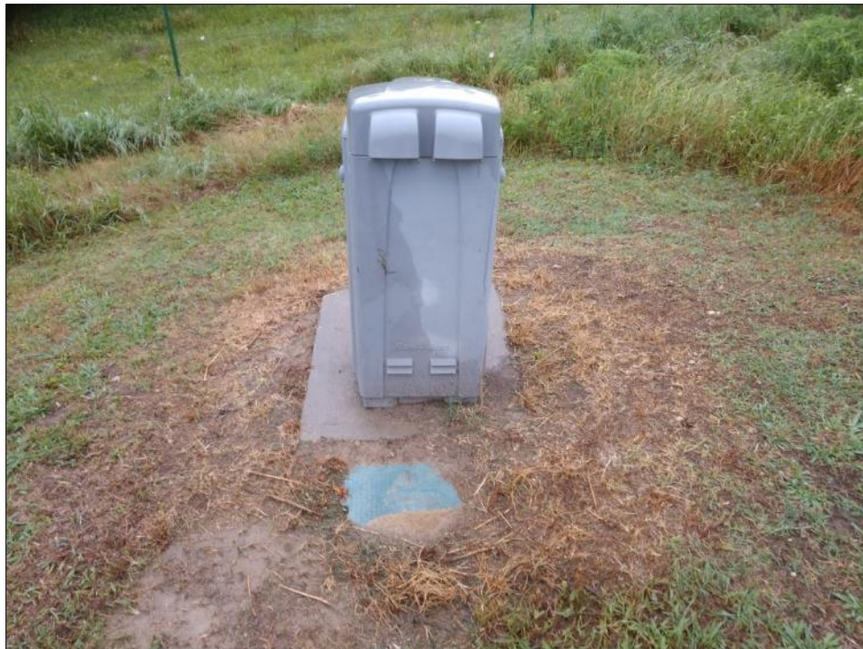
Figure 13. Sprinkler line within Disturbed Area 2.
