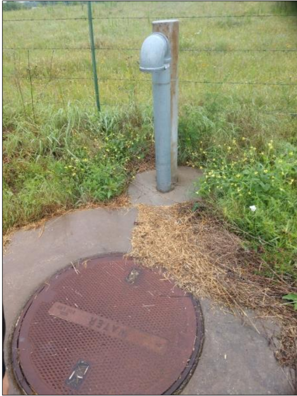
Figure 14. Water line within Disturbed Area 2.
