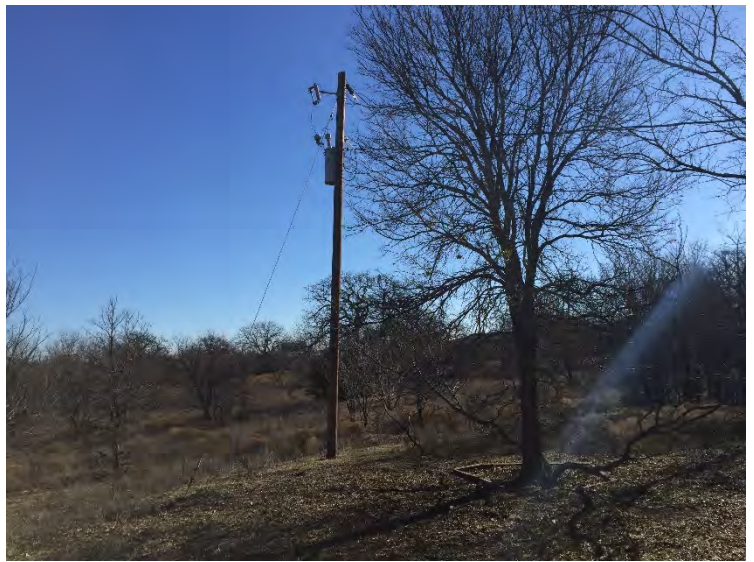
Photograph 20: 41HD96, standing utility pole, facing South.
