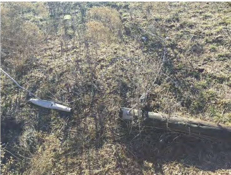
Photograph 17: Site 41HD96, fallen utility pole, facing East.
