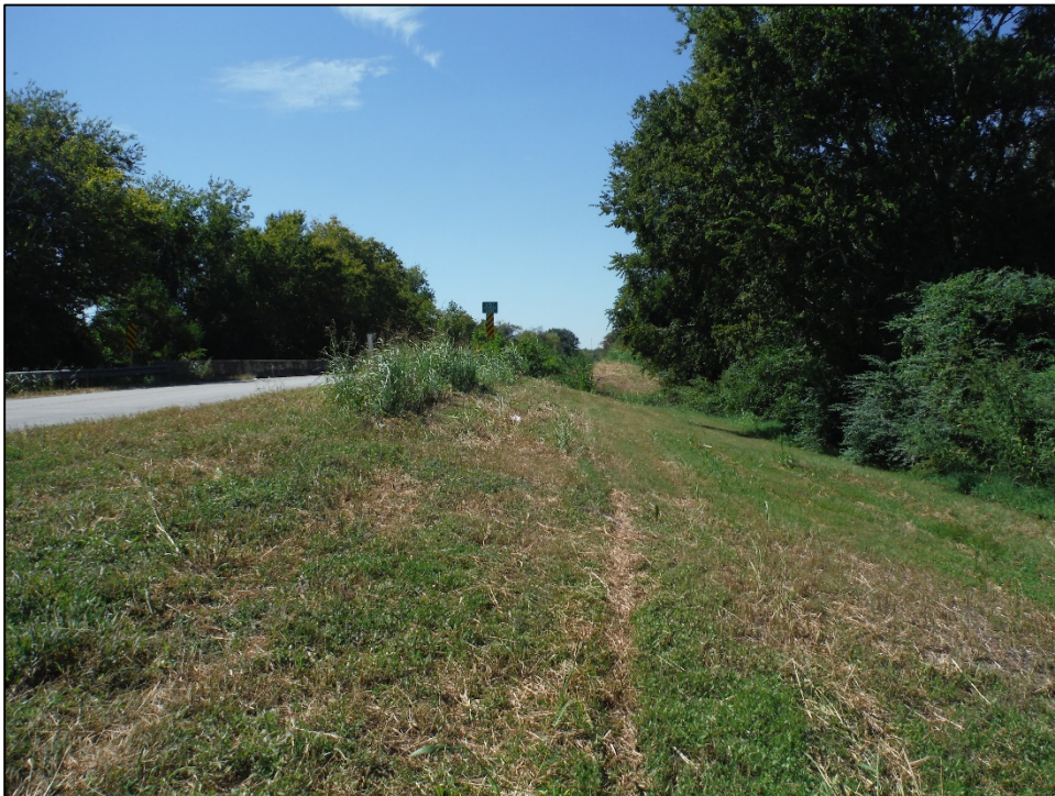
Figure 5-3. Overview of northern shoulder of Bauer Hockley Road within APE gradually sloping upward; facing west.
