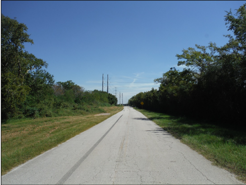
Figure 5-2. View along centerline of APE at the western end; facing east.
