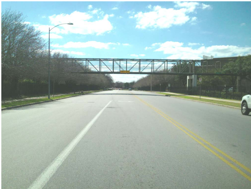
Figure 9: Overview of urban setting of proposed alignment along Alvin Devane Blvd., facing south towards SH 71.
