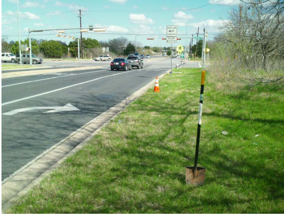
Figure 5: Overview facing north towards the project's northern terminus at the Intersection of East Riverside Dr. and Grove Blvd.
