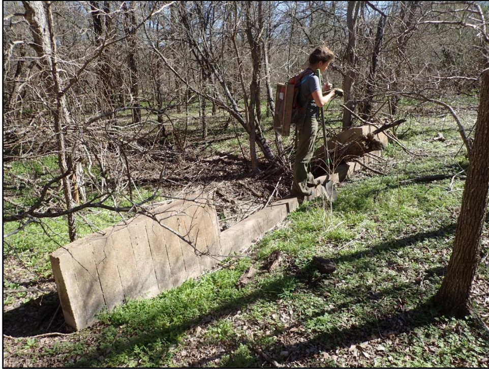
Figure 31. Overview of eastern check dam at site 41TV2526, camera facing southeast.
