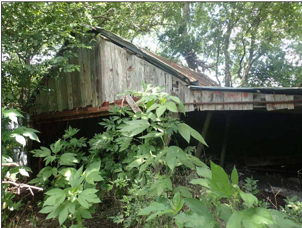
Figure 25. Board and batten garage at site 41TV2524, camera facing north-northwest.
