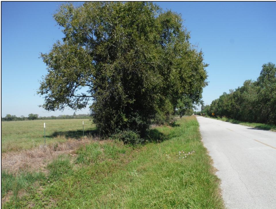
Figure 5-3. View of western shoulder of APE at the northern end; facing north.
