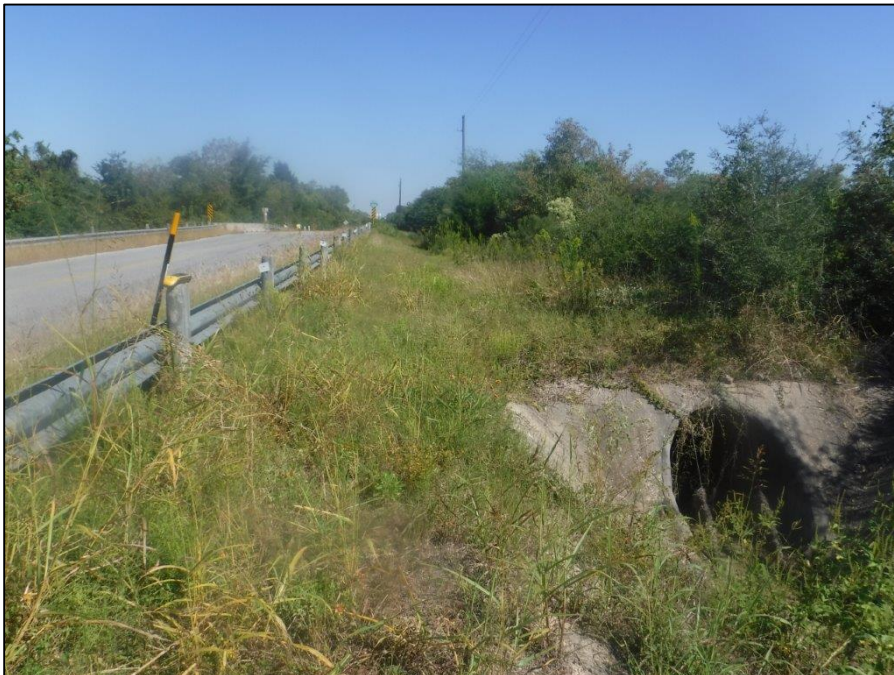
Figure 5-5. No dig shovel test at CM5; facing north.
