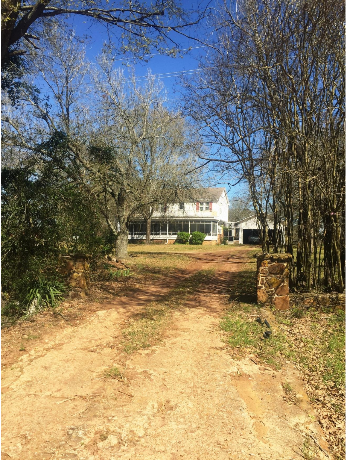
Figure 7. Structure near ST 71 and ST 72 on Segment 3, looking north.
