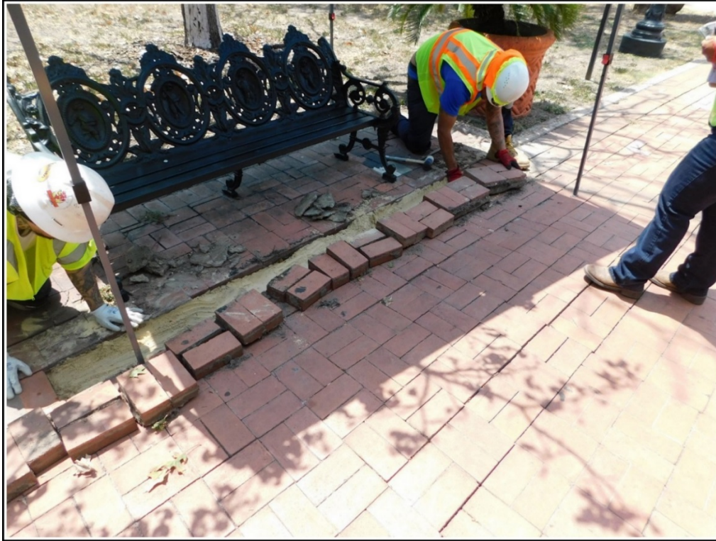
Figure 3-2. Paver repair on the west end of the park facing San Saba Street.
