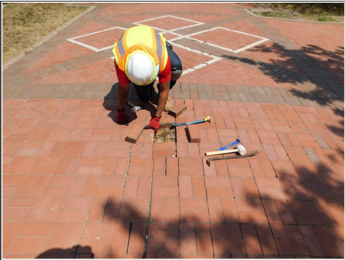
Figure 3-1. Removal of pavers on the west side of the Benjamin Milam monument.
