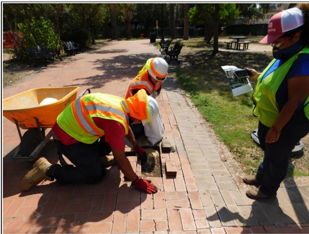
Figure 3-3. Paver repair near the gazebo and playground.
