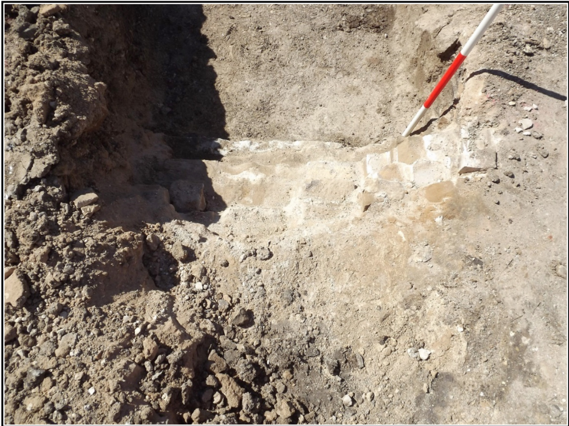
Figure 6-19. An overhead view of the brick foundation comprising 41BX2346.
