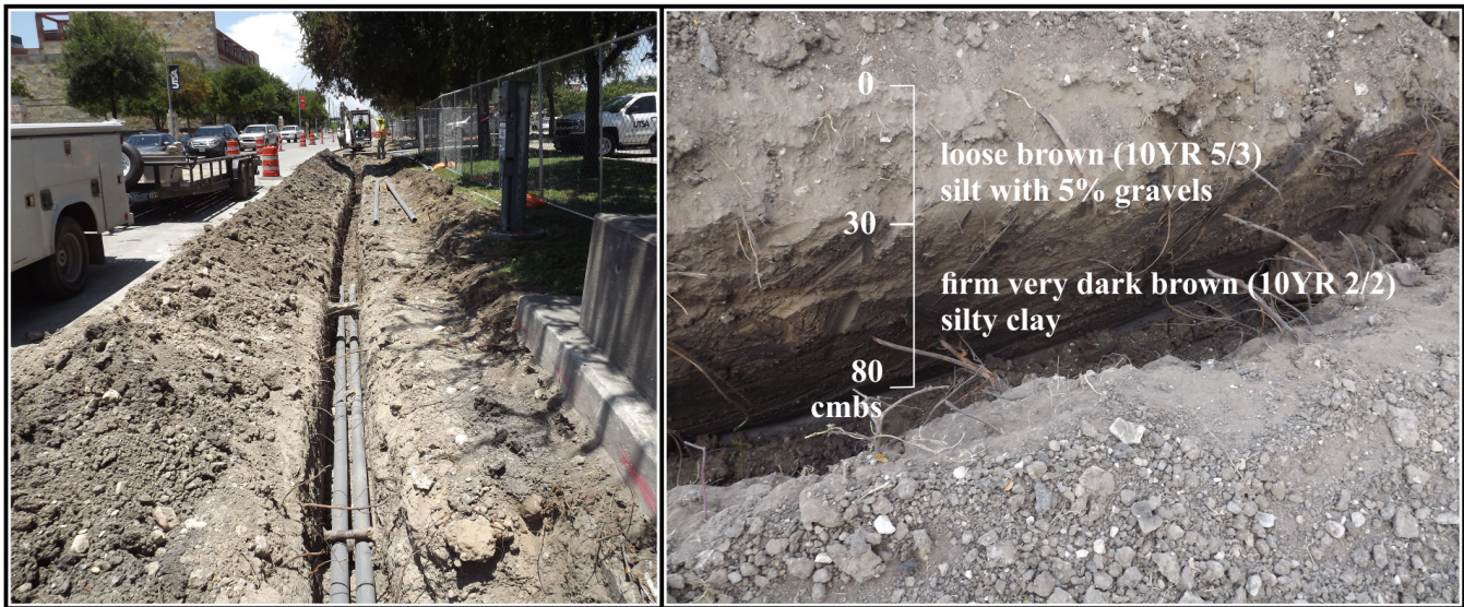
Figure 6-2. Trench 1 excavated on the north side of Buena Vista Street (left). Profile of the southern trench wall (right).
