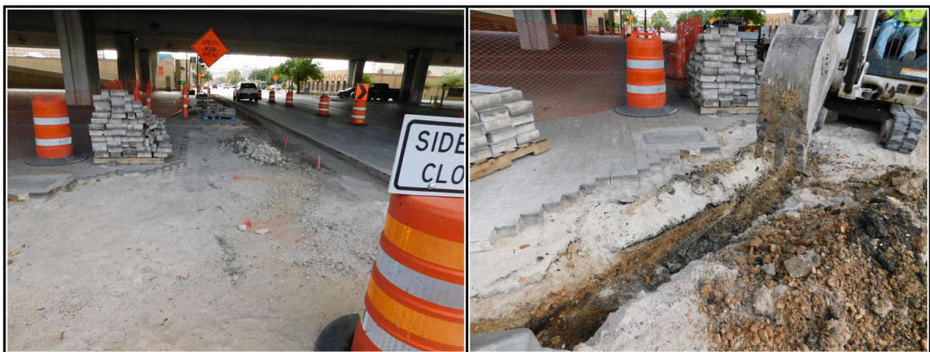
Figure 6-3. The image on the left shows the layout of the trench under the Pan Am Expressway. The image on the right shows the profile of the northern trench wall.
