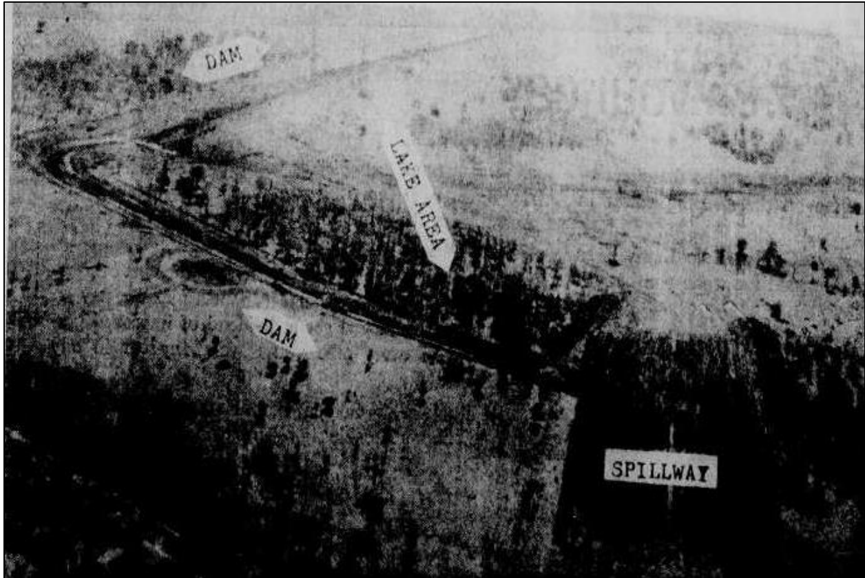
Figure 23. Historic photo, looking southeast, showing Dam No. 9 under construction (Taylor Daily Press 9 March 1959)
