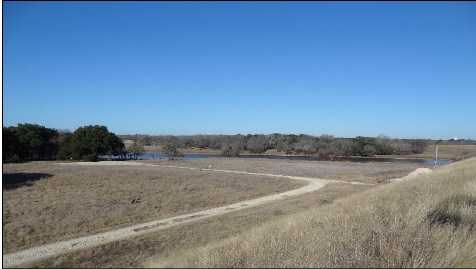
Figure 8. Overview of Dam No. 9 area, facing north
