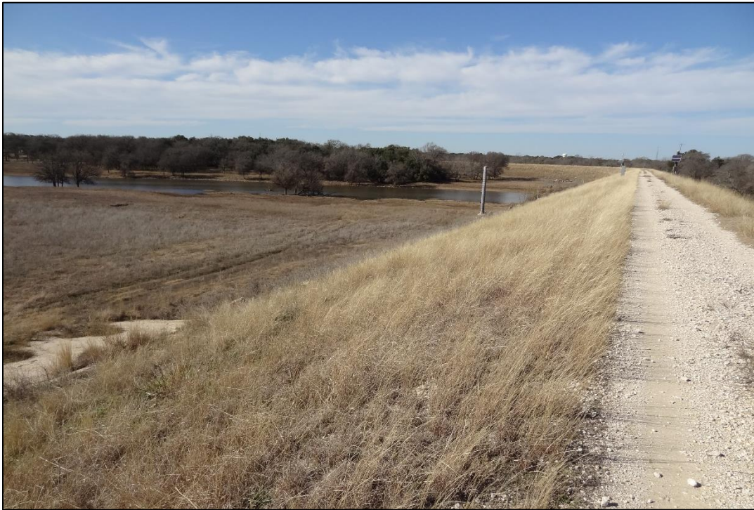
Figure 25. View of Dam No. 9 and inundation lake, facing north
