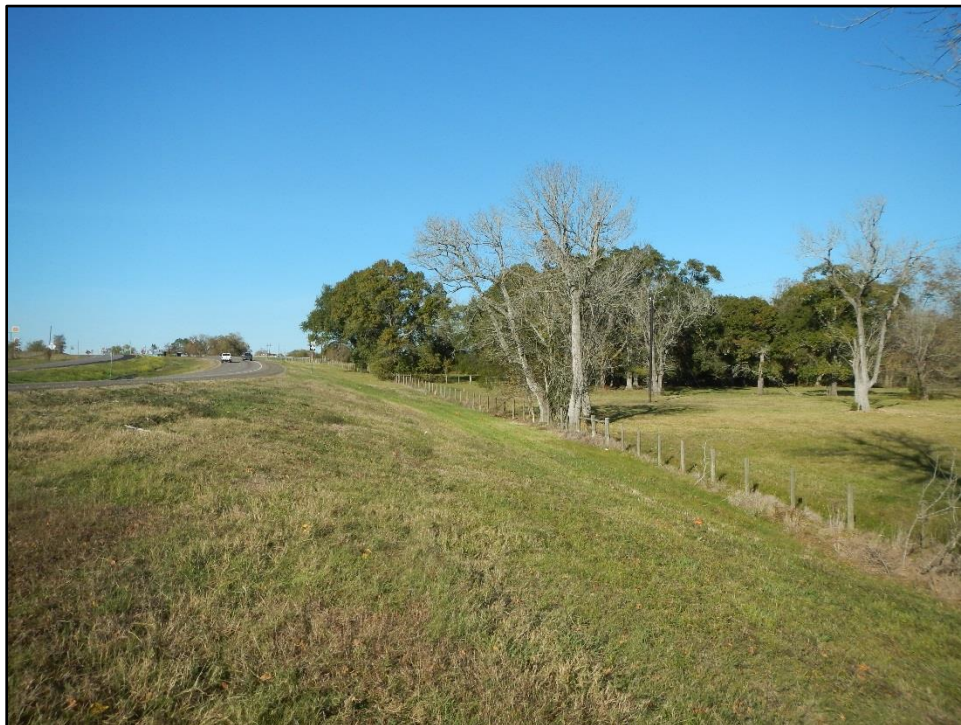
Figure 6. Overview of APE within existing and proposed ROW southeast of SH 6 and FM 2 intersection from just north of Beason Creek, facing north. Note disturbances such as buried and overhead utilities and substantial fill section.
