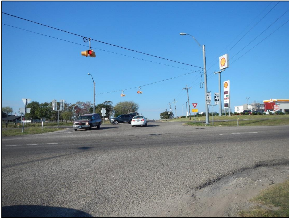
Figure 9. Overview of SH 6 and FM 2 intersection, facing west. Note extensive disturbances and modifications to the area.
