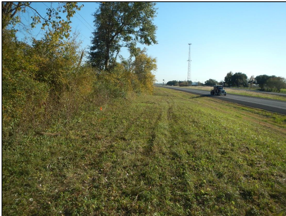
Figure 20. Overview from IF01 at shovel test MG01 within existing ROW along northeastern margin of APE severely sloping down toward ditch and roadway, facing southeast.
