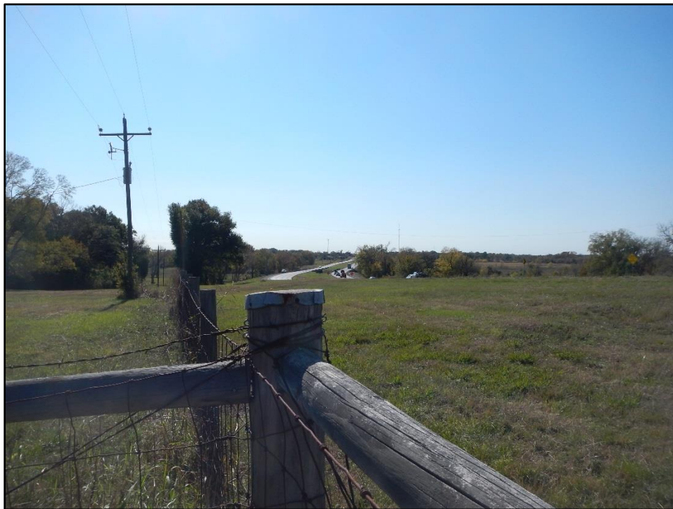
Figure 15. Overview of side-by-side bridges along SH 6 over Beason Creek from Parcel 11789 (Double H Ranch) within proposed ROW, facing southwest.
