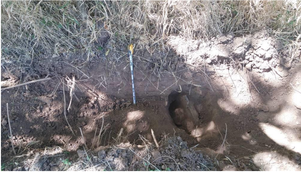
Photo #9: Relatively large existing wastewater line exposed in BHT 2.
