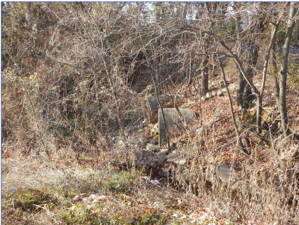
Figure 6. Drainage culverts under rail spur berm; view south.
