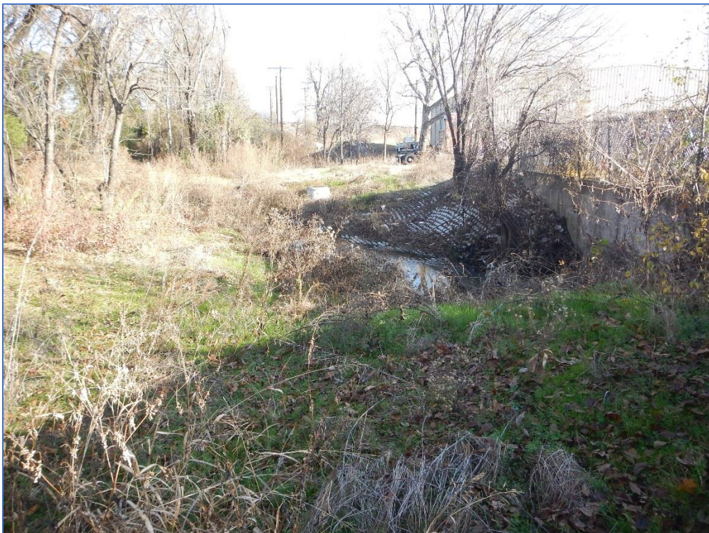
Figure 10. Erosion control measures behind truck yard fence in northeast corner; view north.
