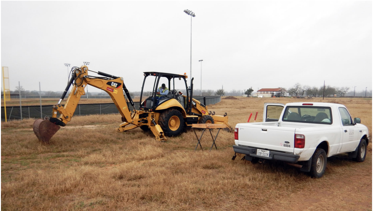
Figure 4. Backhoe and operator beginning excavation of trench BT1.
