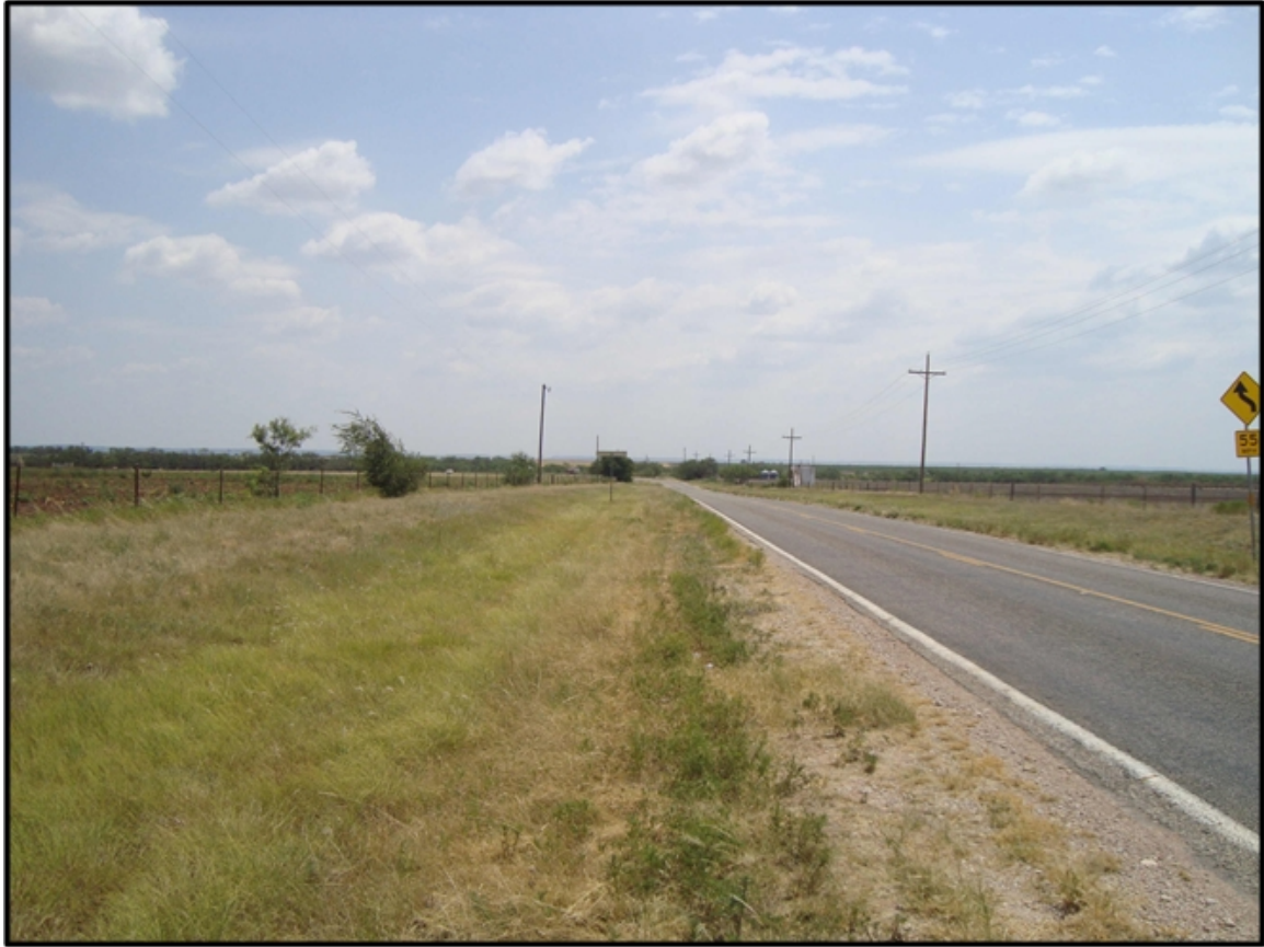
Transmission Line on North Side of Ranch Road 1770
