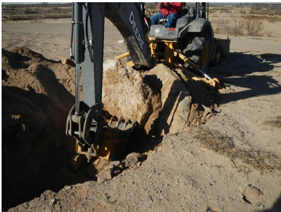
Figure 12. Large concrete slab section being removed from BHT 3.
