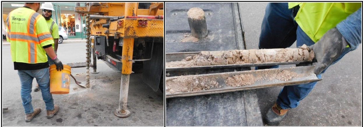
Figure 4-3. B-1: left) boring in progress, view southeast, and right) first core sample.
