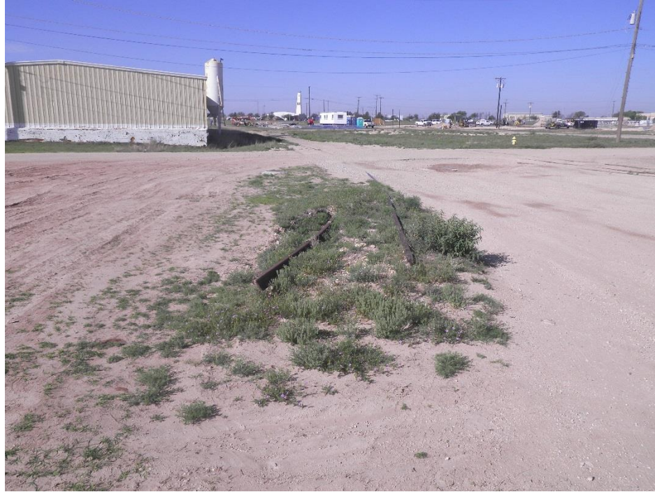
Figure 11. View west from northeast end of APE, along proposed roadway route and current route of historic-age railroad track remnants. Note that rails are partially buried in the background and pulled up/misaligned in the foreground.
