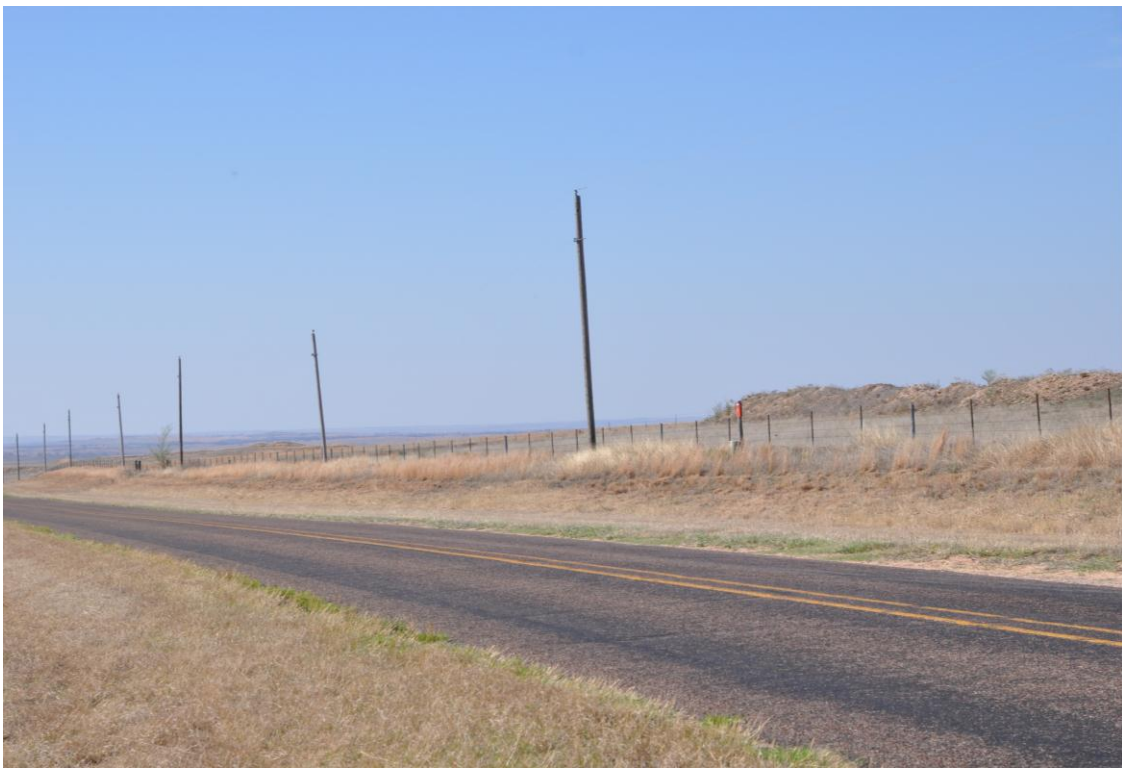
Figure 8. West side of FM 48 at 41WE20. Note: steep grading and utilities.
