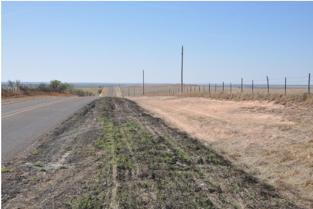
Figure 9. West side of FM 48 at 41WE20. Note: recent steep grading.
