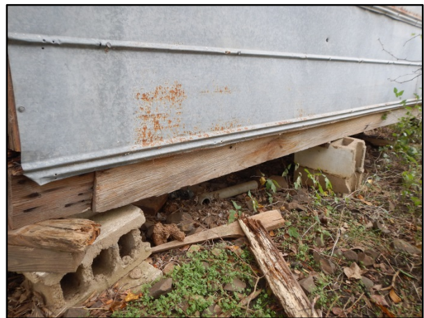
Figure 7. Cinder blocks and wooden blocks under barn, facing southwest.
