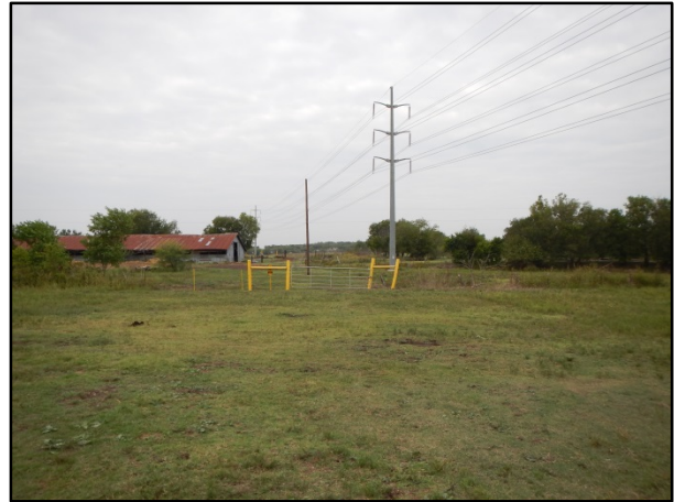
Figure 5. Overhead utility and buried pipeline crossing APE, facing northwest.
