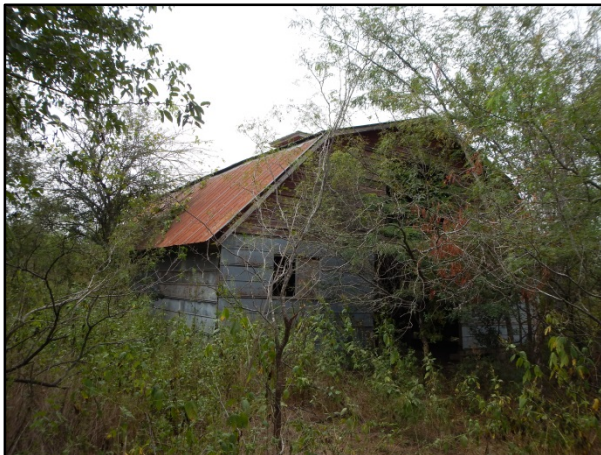
Figure 6. North façade of barn, facing southwest.
