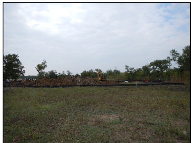
Figure 8. Active construction in site 41TV2366, facing southwest.
