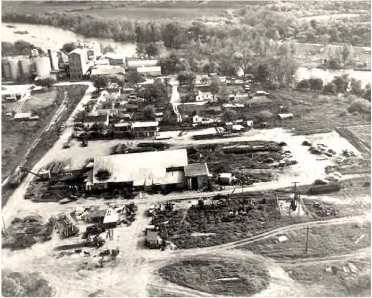
Figure 17. Photo looking west at 4 th Mill Seguin Milling and Power company (located 3.5 miles west of the Courthouse at Erskine's Ferry; Guadalupe River in background).
