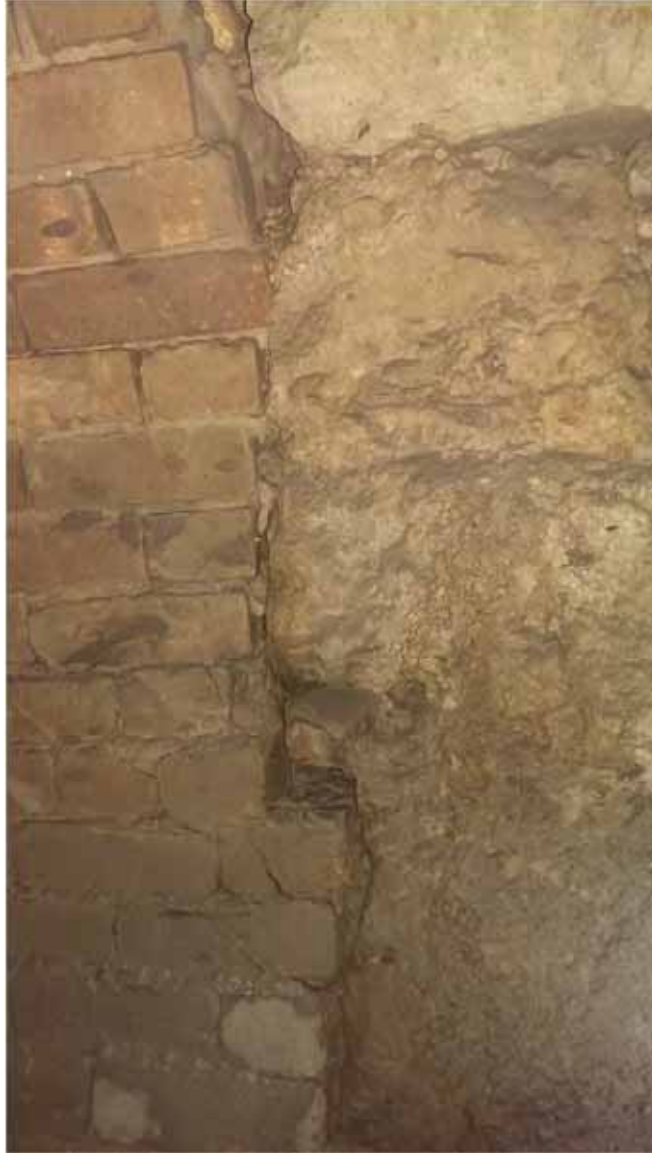
Figure 2. Connection between conglomerate and brick masonry tunnel wall (VPS 2015).
