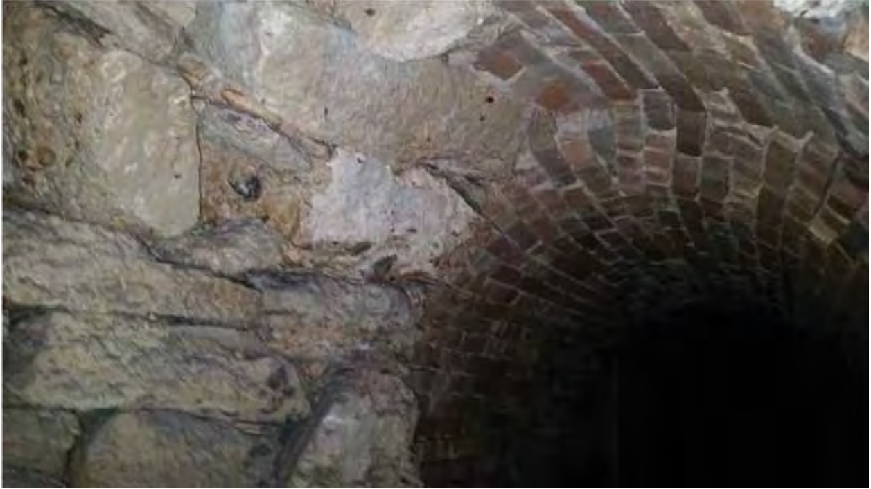
Figure 7. View of Rubble brick course transition in culvert, looking south.
