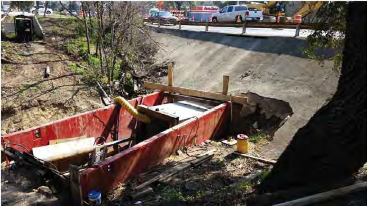
Figure 4. View of culvert installation under E. Court St, looking southeast.
