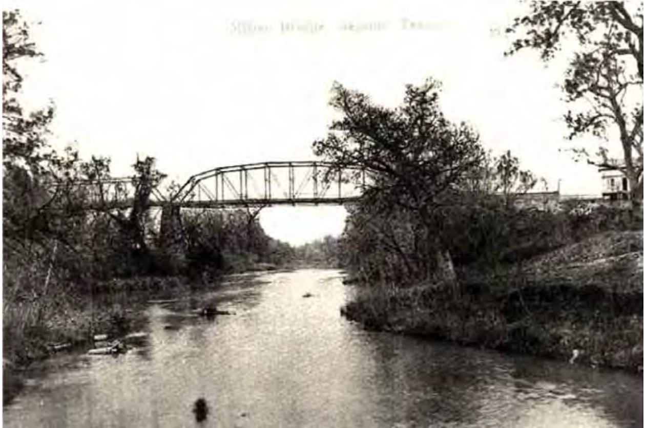
Figure 15. Miller Bridge at the 2 nd Mill location Seguin Electric Light and Water Company Power Plant.
