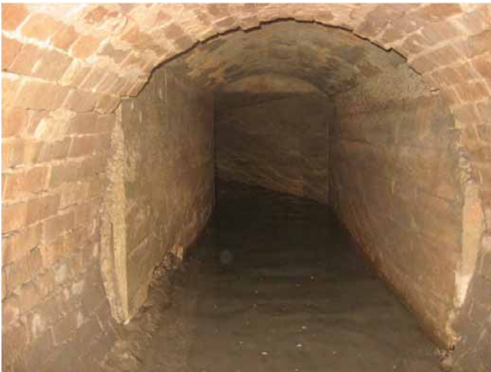
Figure 10. View of modification of southern end to accommodate box culvert (ca. 1925-1930).
