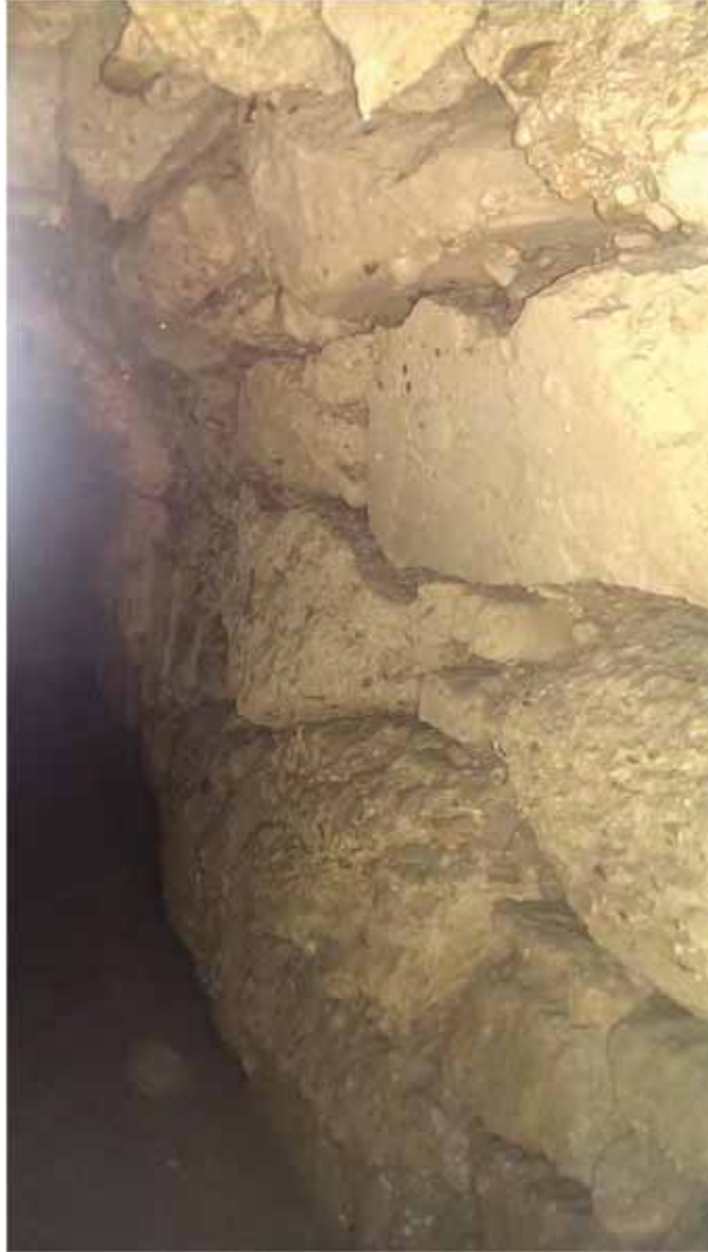
Figure 1. View of rough-cut stacked conglomerate at west wall of tunnel (VPS 2015).
