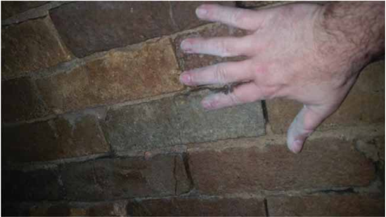
Figure 8. View of brick course on western side of culvert.
