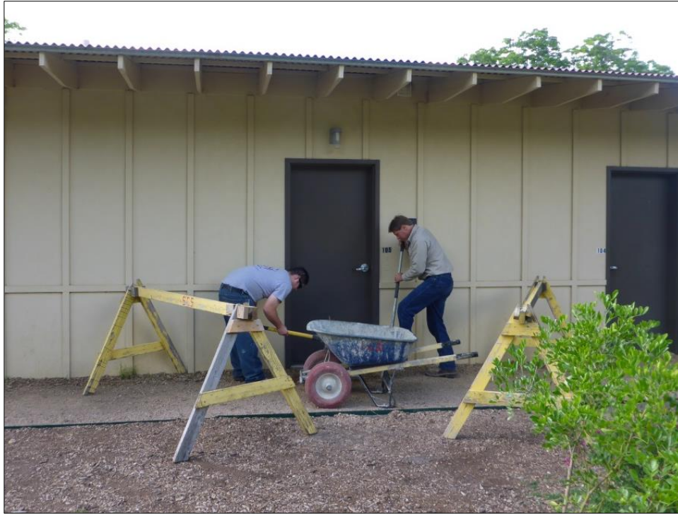
Figure 17. Small-scale manual excavation for ADA upgrades at the MCWE Ticket Kiosk building.
