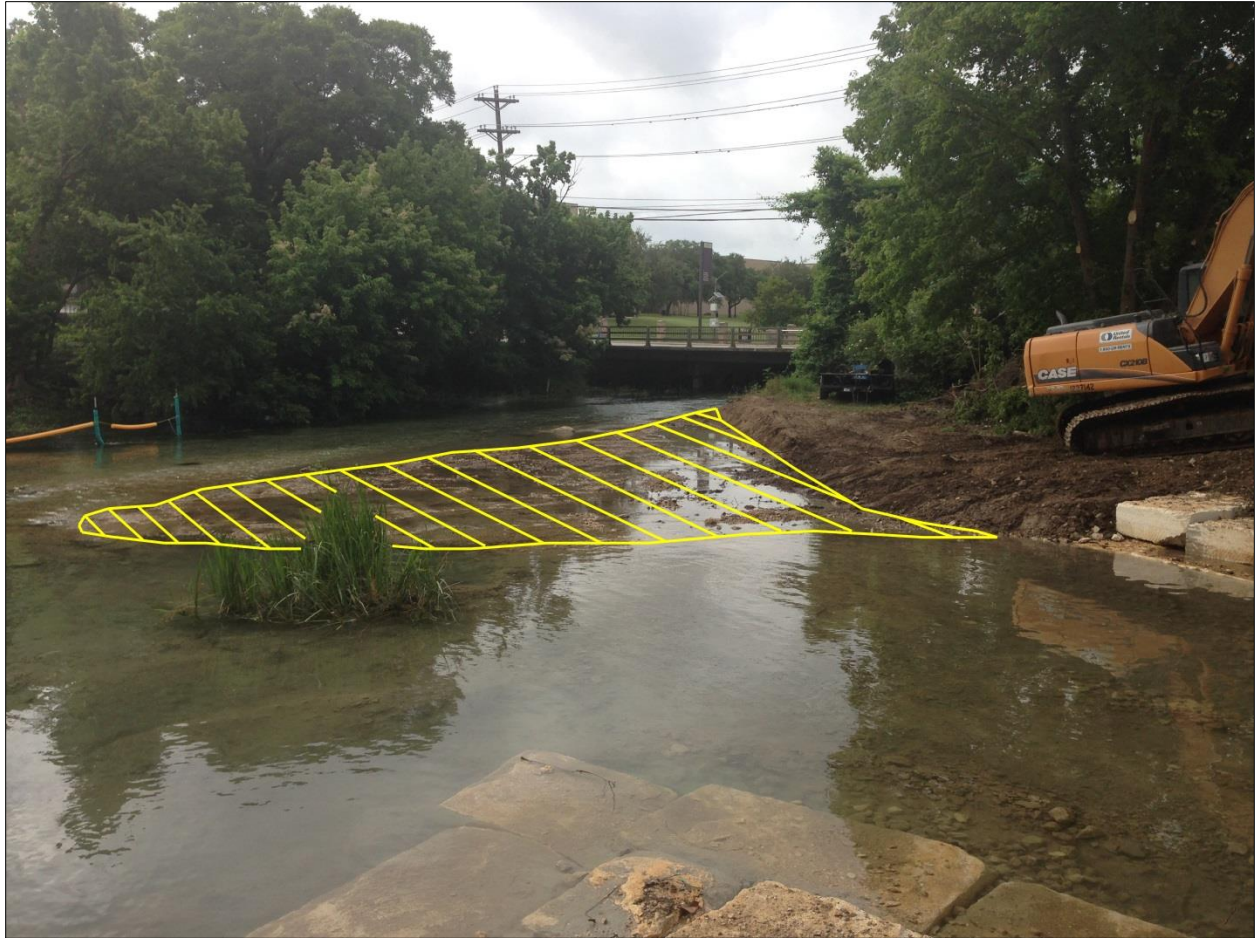
Figure 33. Highlighted area where a small peninsula on south side of the confluence of Sessom Creek and the San Marcos River was excavated down to water level.
