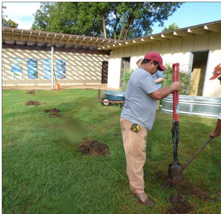
Figure 18. Post hole excavations for Divers Yard fence installation at Spring Lake.
