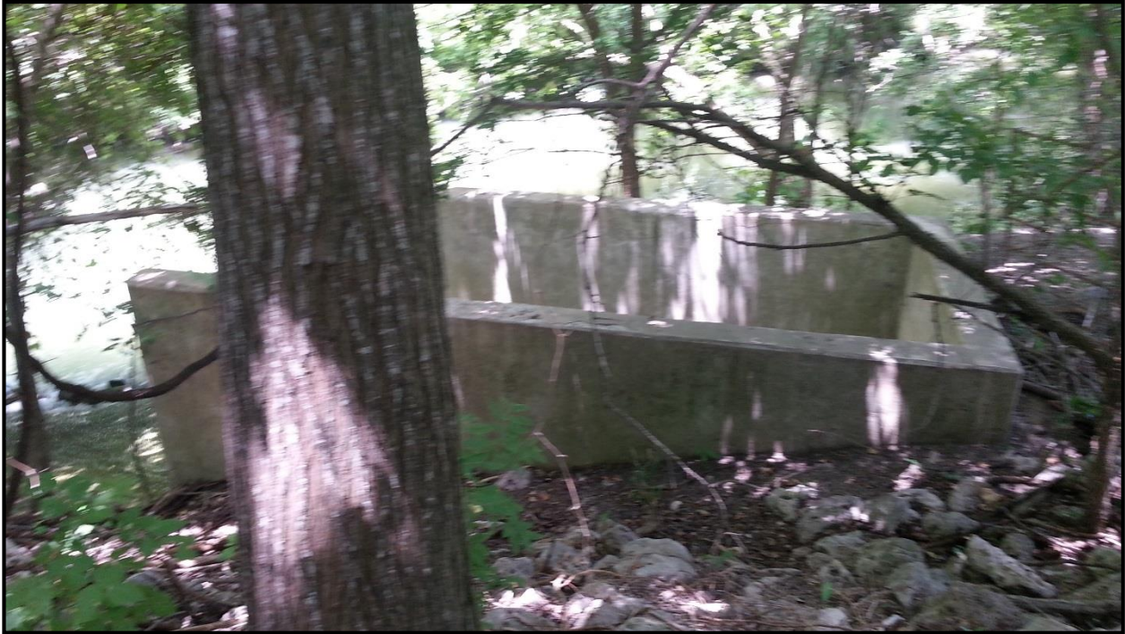
Figure 1-4. Existing outfall structure on eastern edge of Geronimo Creek that will be abandoned in place (photograph by Todd Schnakenberg).
