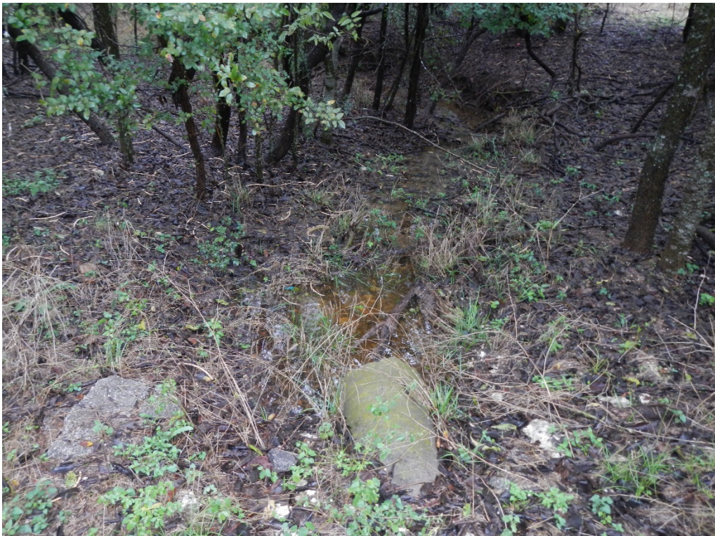
Figure 10: View of small culverted drainage in APE. Facing northwest.
