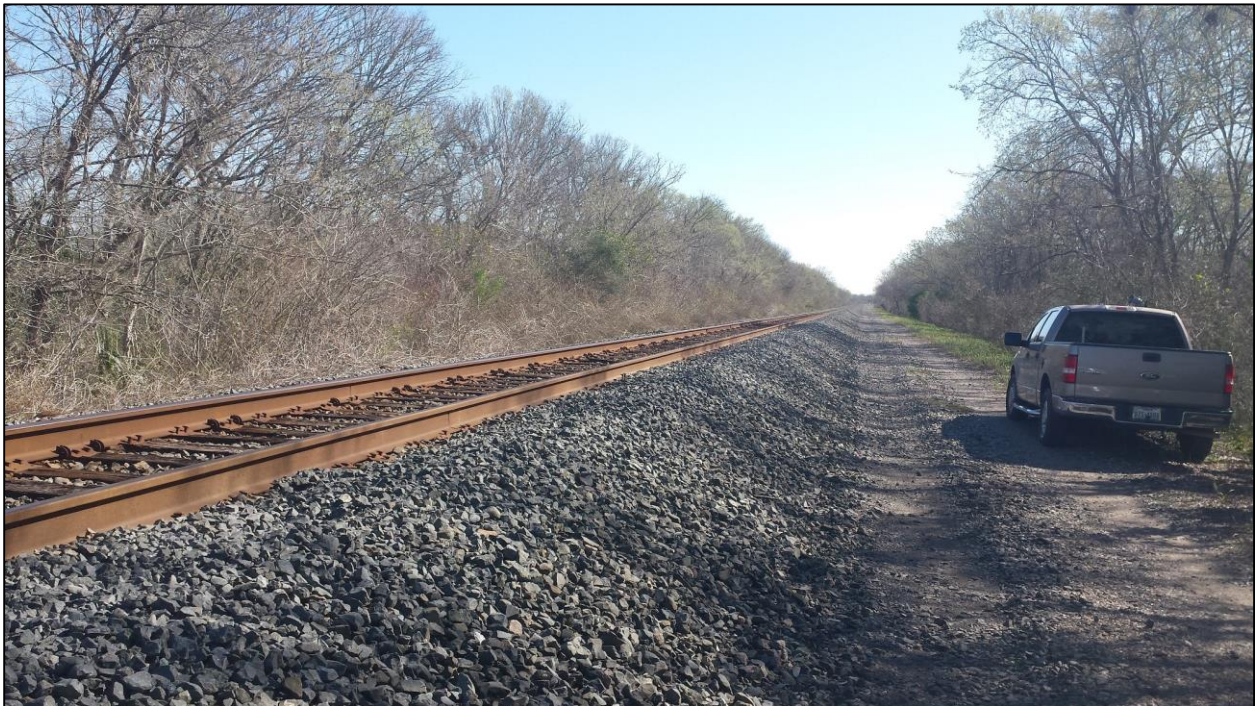
Figure 8. Overview of the existing railroad along the northern boundary, facing east.
