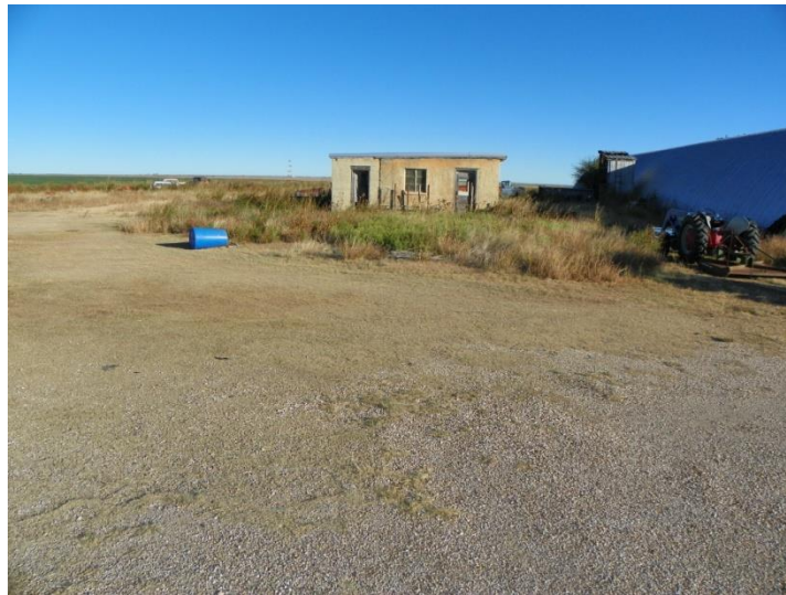
Scales Building, looking North (note elevator cowling next to modern barn)
