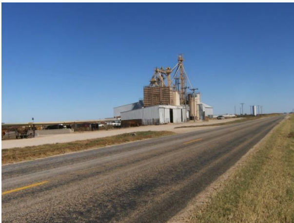
Tulia Feed Lot along Segment 5
