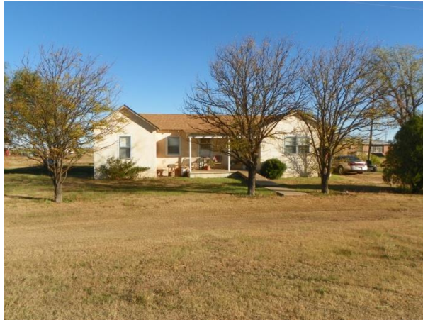
Last Older Building Still Occupied facing North
