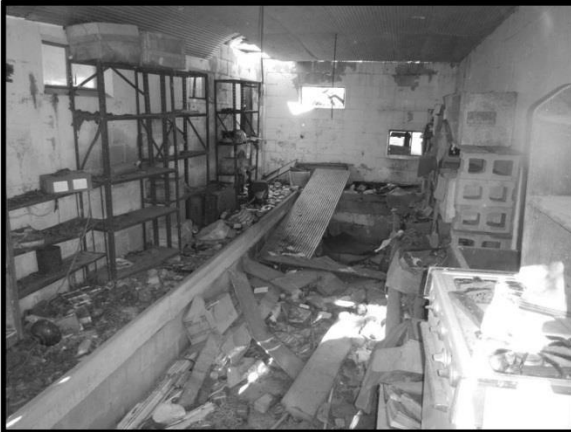
a. View of Milking Room Interior Facing North.
