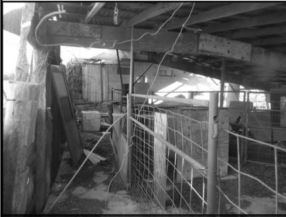
c. View of Covered Pen Interior Facing East
