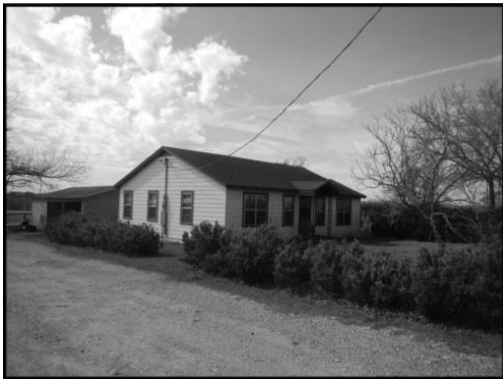
Figure 9. View of 1947 House Facing Southwest
