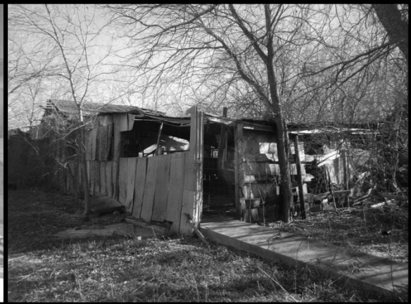
b. View of Covered Cattle Pen and Walkway Facing East
