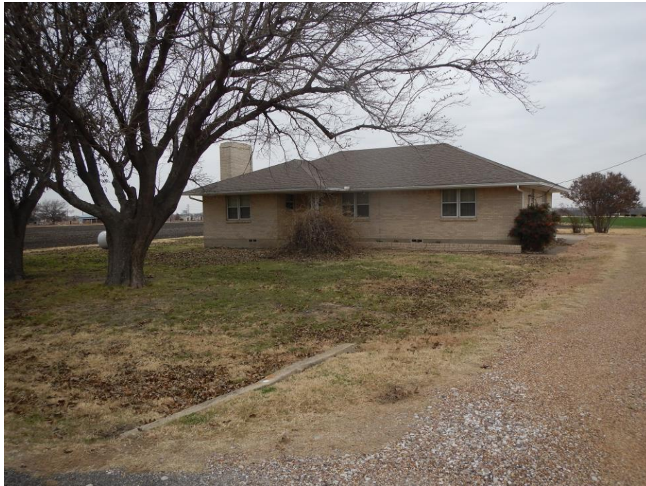
Figure 9. Small Ranch-style residence (Structure C) facing Witt Road; looking north northwest
