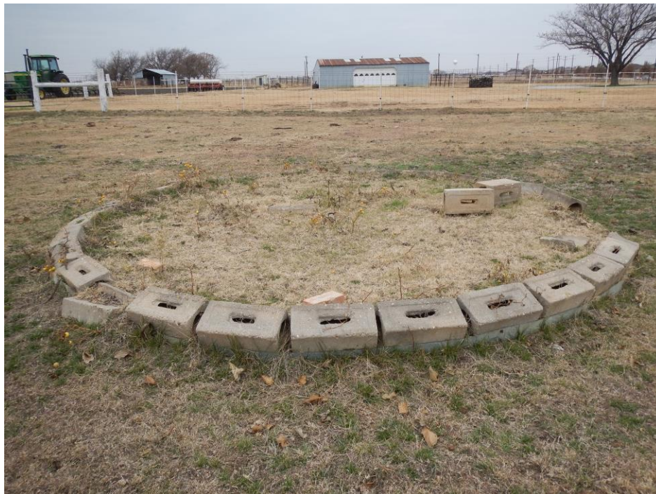
Figure 4. Concrete block silo foundation; facing west
