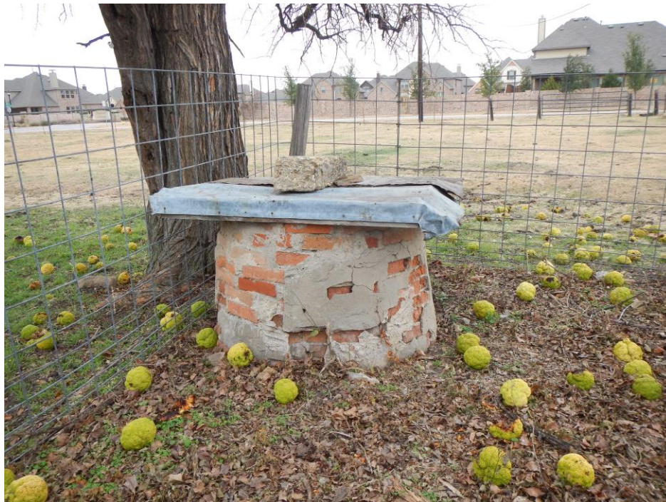
Figure 13. Above ground portion of the original well/cistern at site 41DN589; facing south
