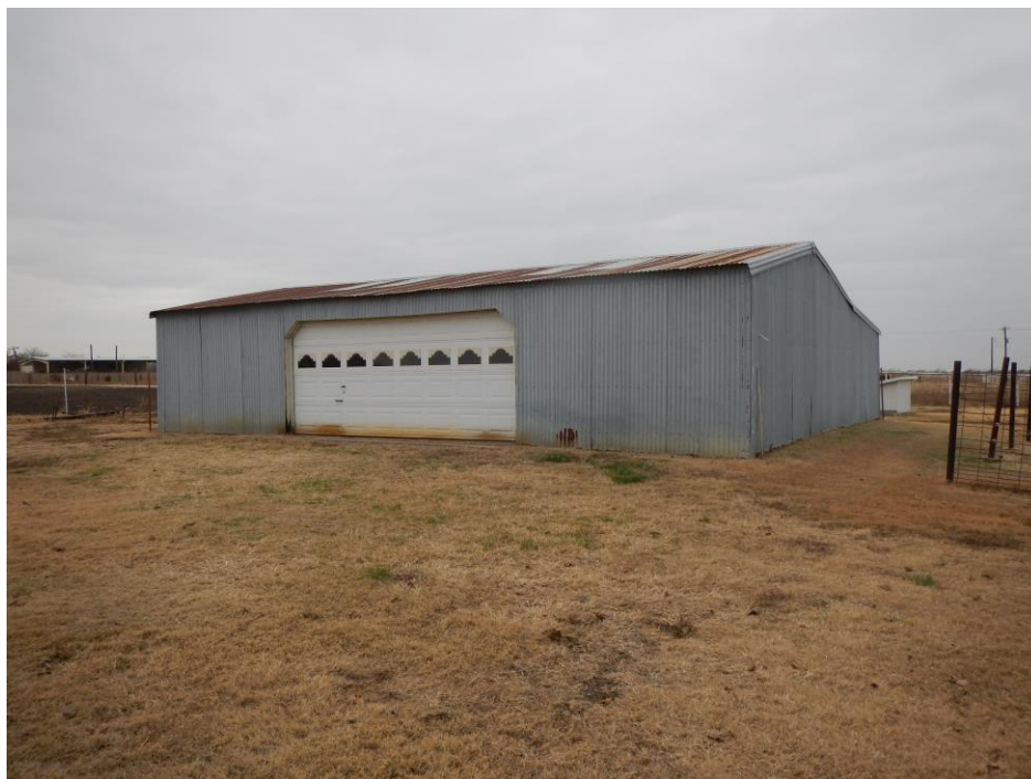
Figure 8. Metal garage (Structure B) servicing King Road residence; facing west
