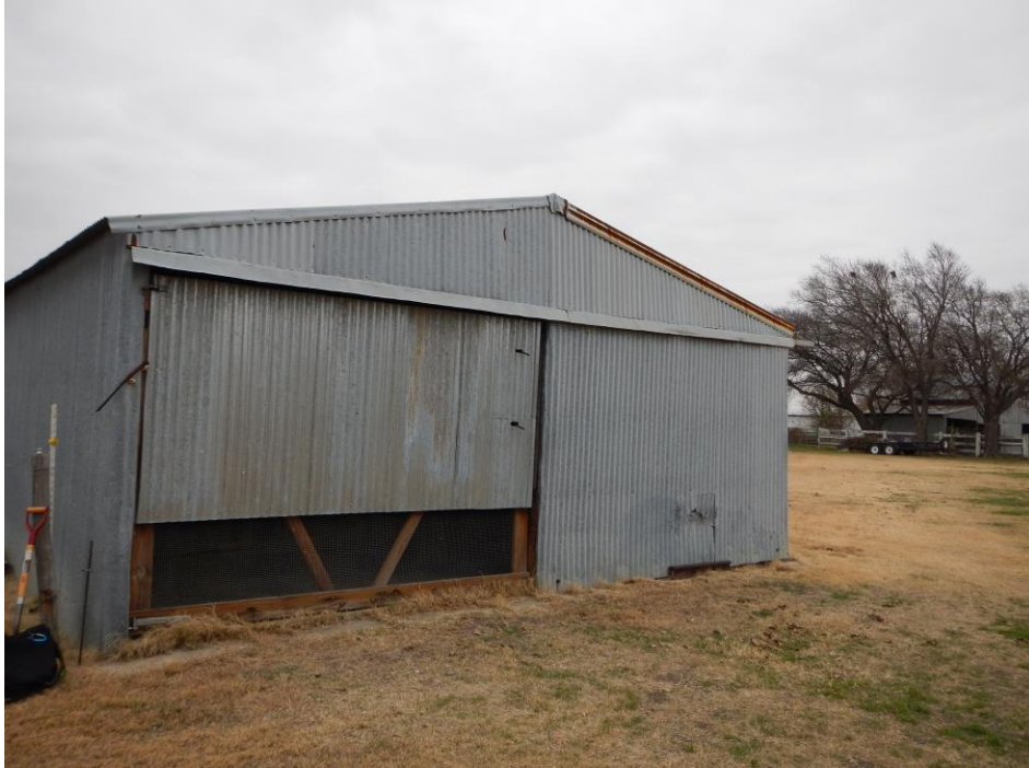
Figure 14. Metal building (Structure D) behind Witt Road residences; facing northeast
